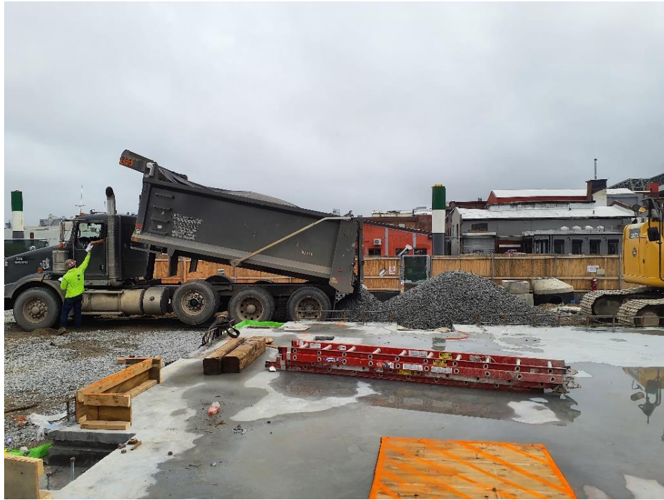
Photo 1: Bauer importing ASTM #5 stone to the site (facing east)
