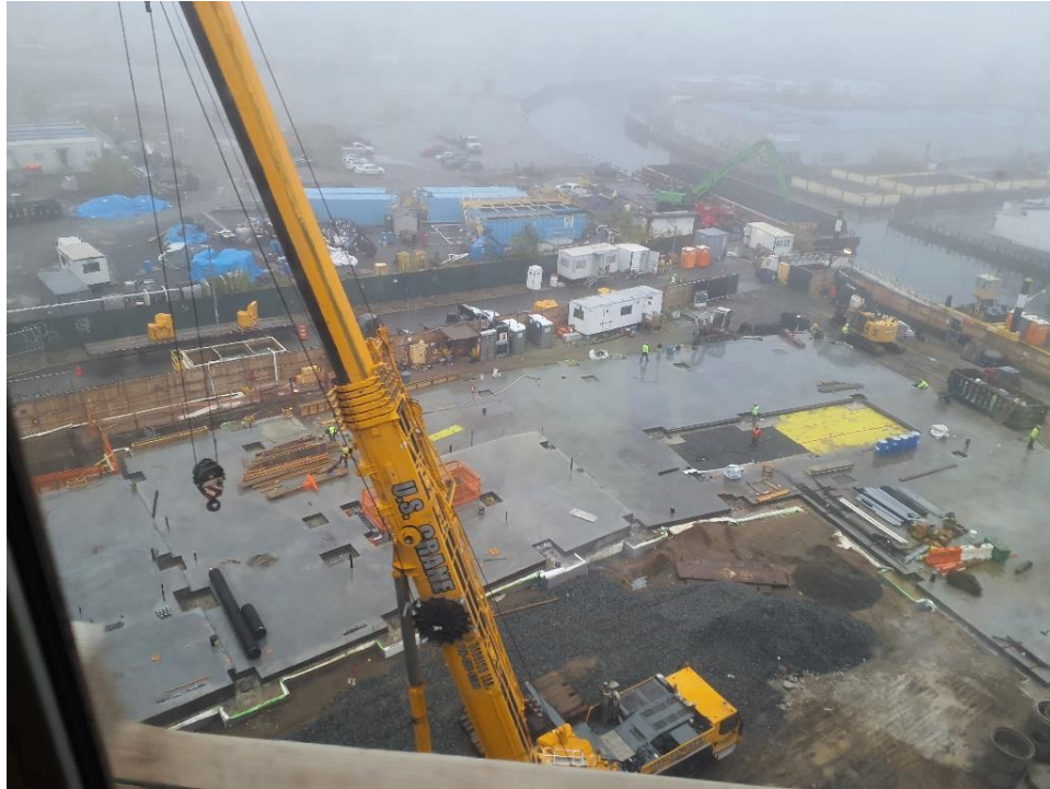
Photo 2: Aerial view of the site condition (facing northeast)
