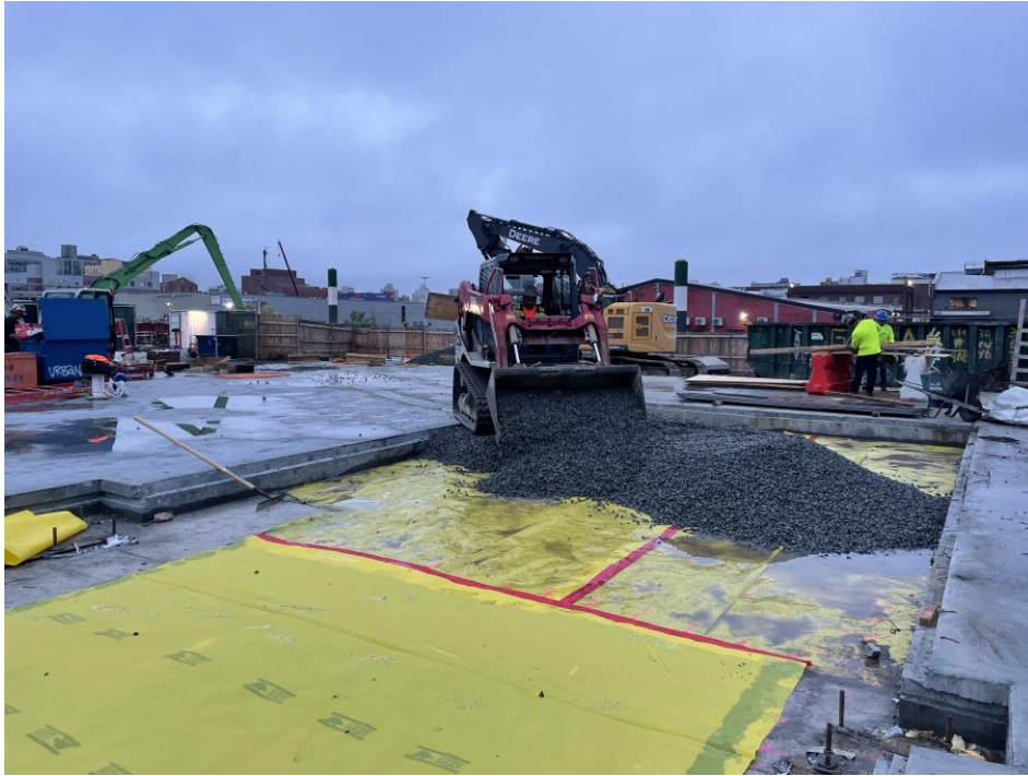
Photo 1: Bauer backfilling with ASTM #5 stone in the eastern part of the site (facing east)
