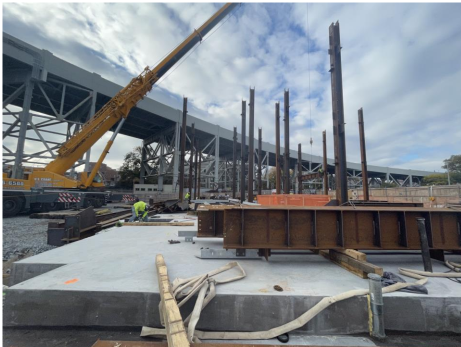
Photo 2: View of the western site condition (facing west).
