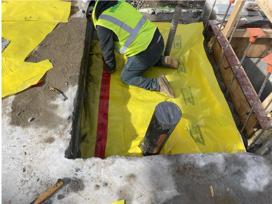
Photo 1: Bauer installing Stego® Wrap 20-mil Vapor Barrier in the western part of the site (facing west)
