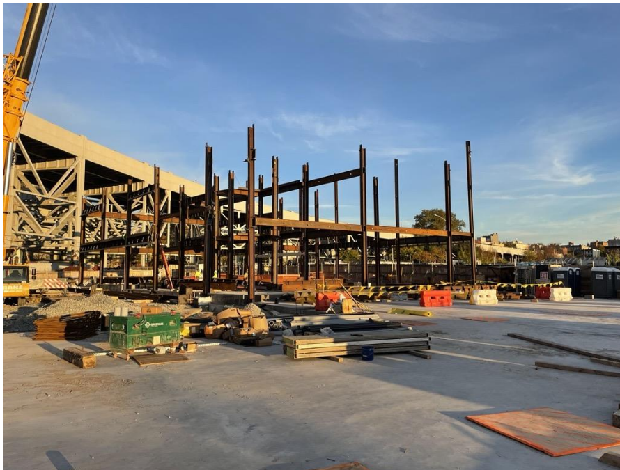
Photo 2: View of the western and central parts of the site (facing northwest)
