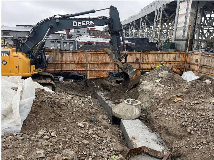
Photo 1: Bauer returning previously excavated fill to the original location in the southeastern part of the site (facing east)
