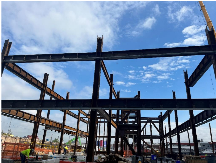
Photo 2: Super structure progress in the central part of the site (facing east)
