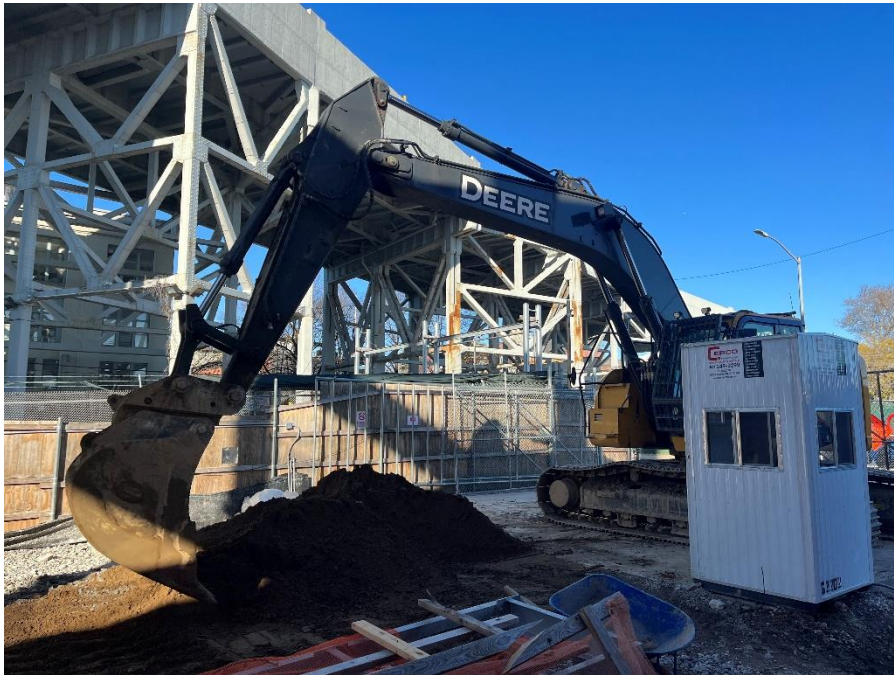
Photo 1: Bauer stockpiling imported clean fill from EROC in the northwestern part of the site (facing northwest)
