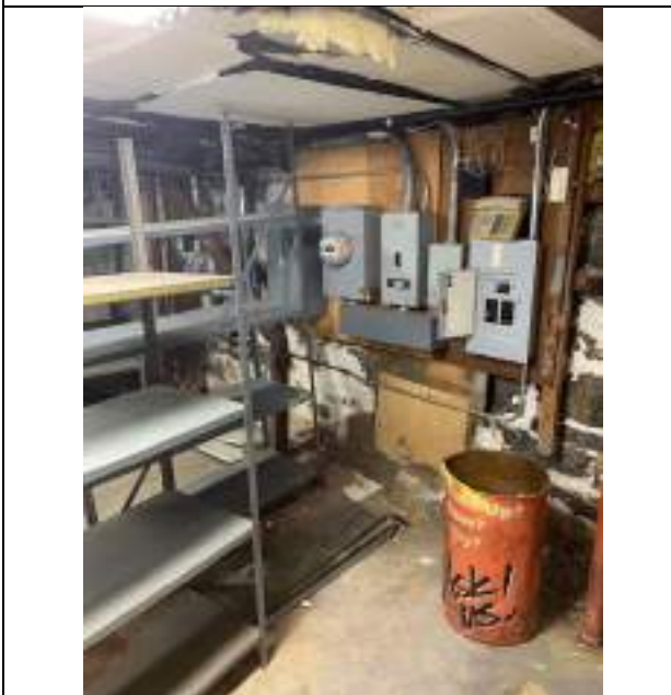
Basement Beneath 1036 with view of utilities and sump pump.
