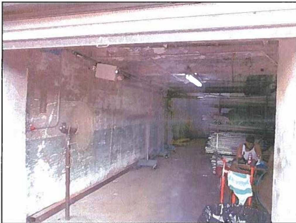
32 : View of the loading bay at 253 Bond Street
