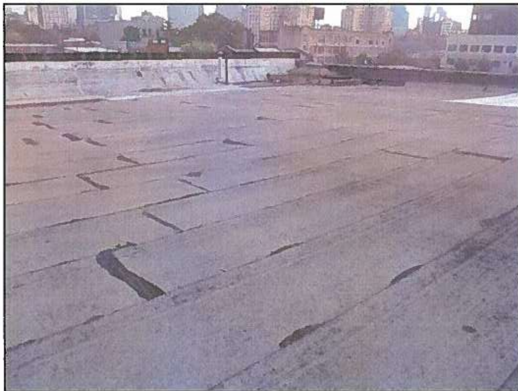
54 : View of the roof at 253 Bond Street.
