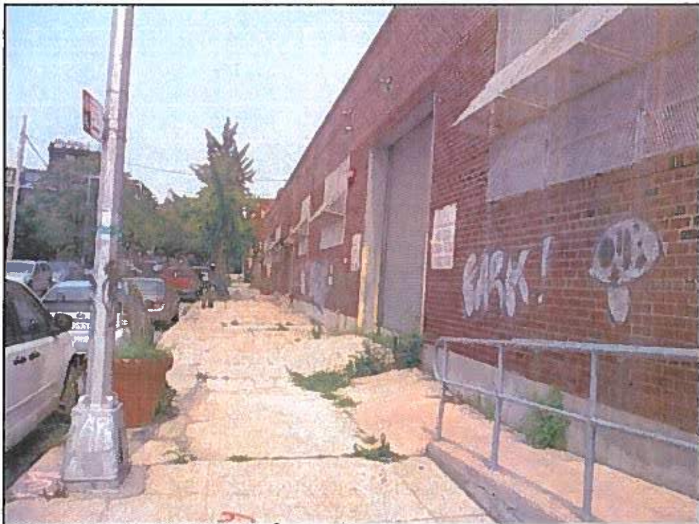
4 : View of the southwestern side of 210 Douglass Street, along Degraw Street.
