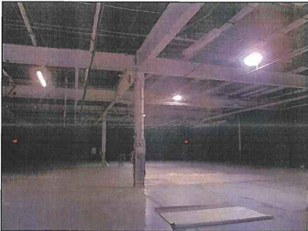
12 : View of the warehouse at 210 Douglass Street.
