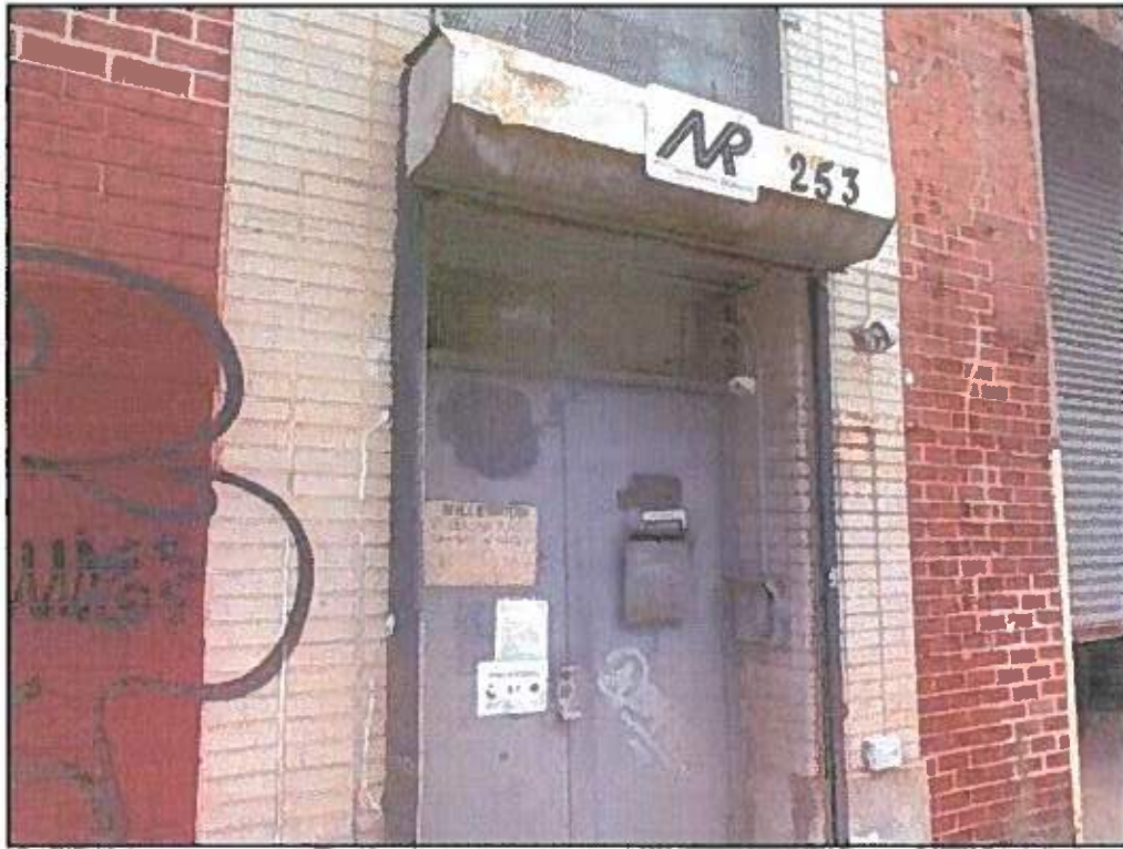
25 : View of the entrance to 253 Bond Street.
