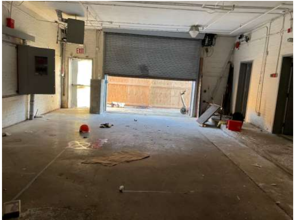
Photo 1 – General Site conditions on Lot 14, facing north.
