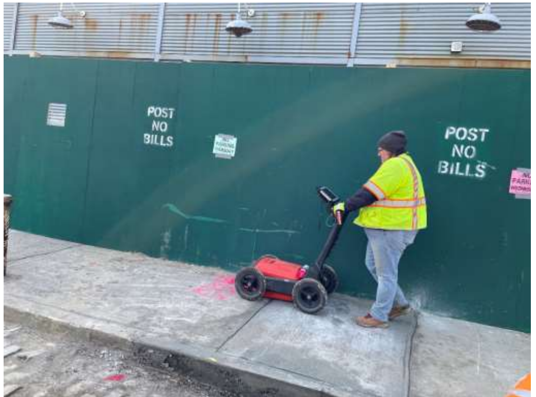
Photo 2 – Hager-Richter clearing sidewalk soil boring location LSB-26, facing south.
