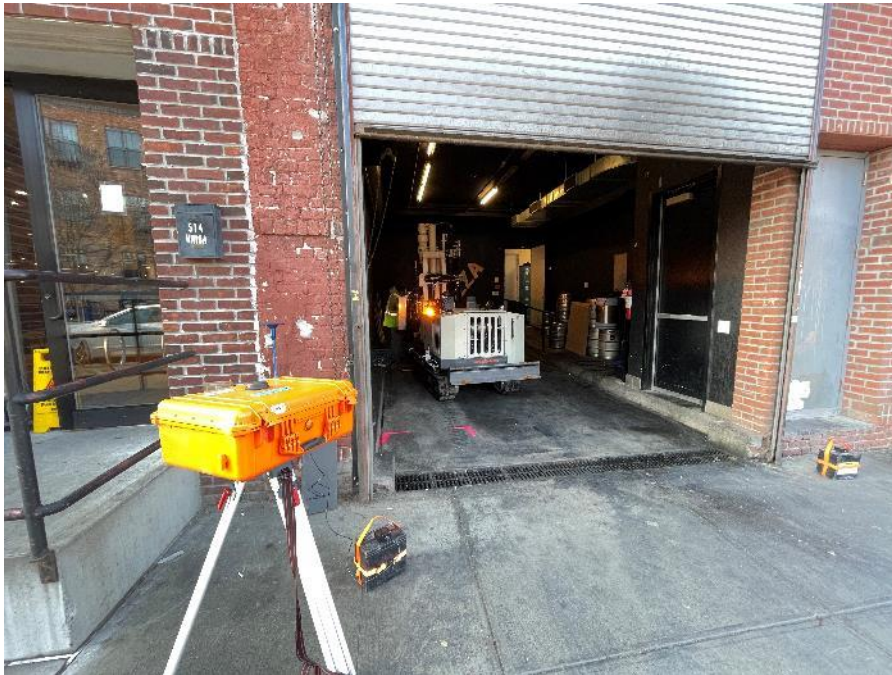
Photo 1: Coastal Environmental installing monitoring well MW15D (facing south).
