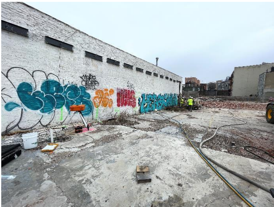
Photo 2: Regenesis applying remedial products at injection point IP-42 (facing east).
