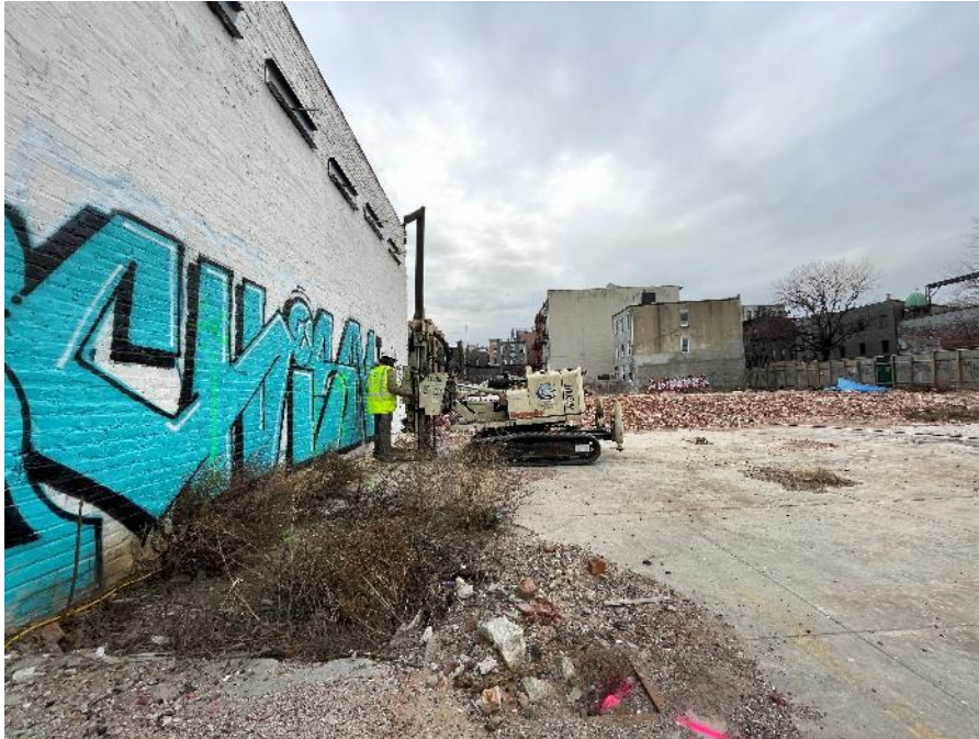
Photo 1: Coastal Environmental advancing soil boring SC-1 (facing east).
