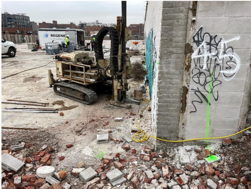
Photo 1: Regeneis applying remedial products at injection point IP43 (facing west).
