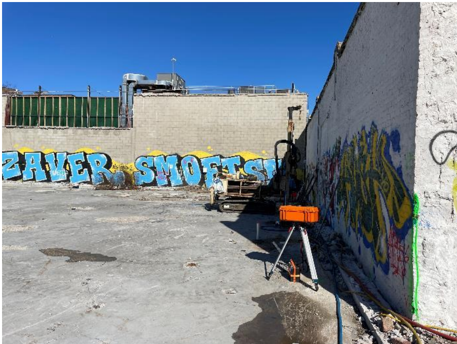
Photo 2: Regenesis applying remedial products at injection point IP09 (facing north).
