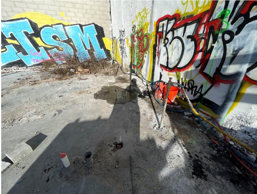
Photo 1: Injection points IP06, IP07 and IP08 (facing northeast).
