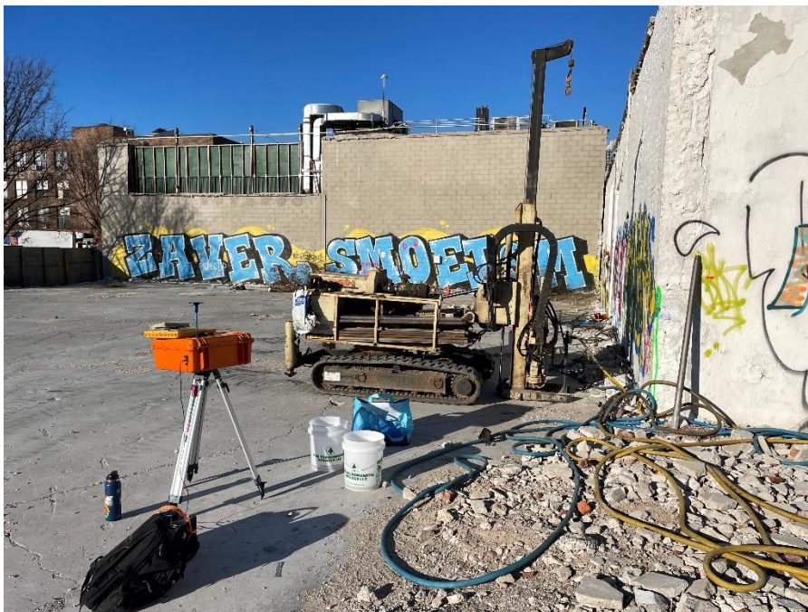
Photo 2: Regenesis applying remedial products at injection point IP14 (facing north).
