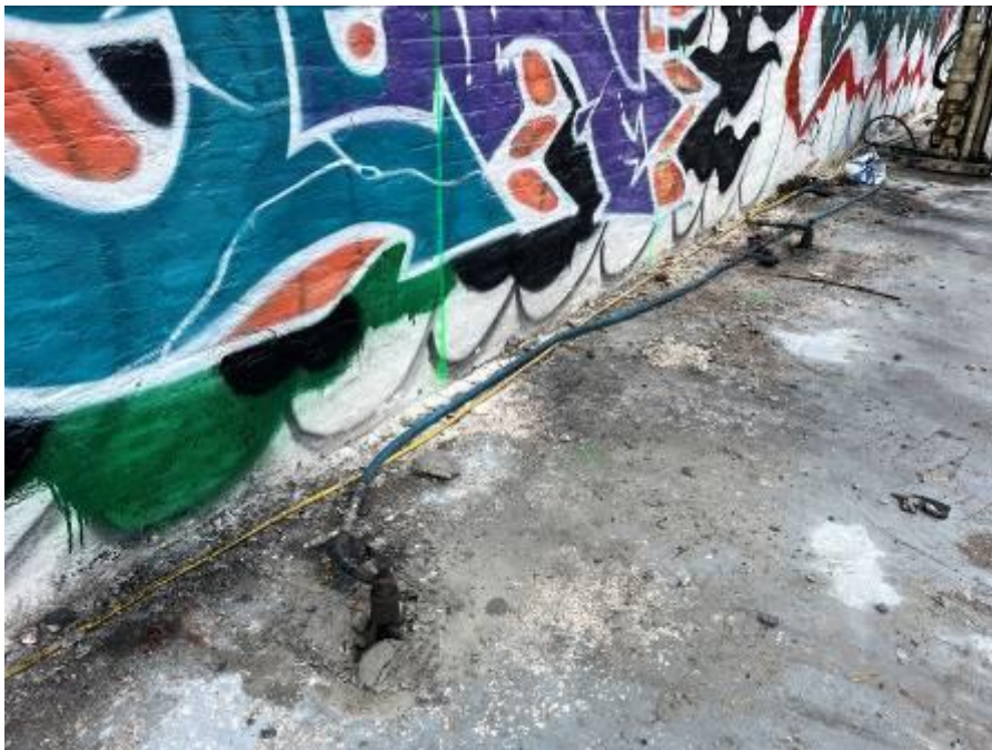
Photo 2: Regensis applying remedial products at injection points IP22 and IP24 (facing northeast).
