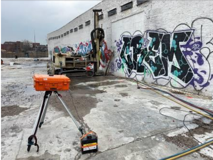
Photo 1: Regensis applying remedial products at injection point IP26 (facing northwest).
