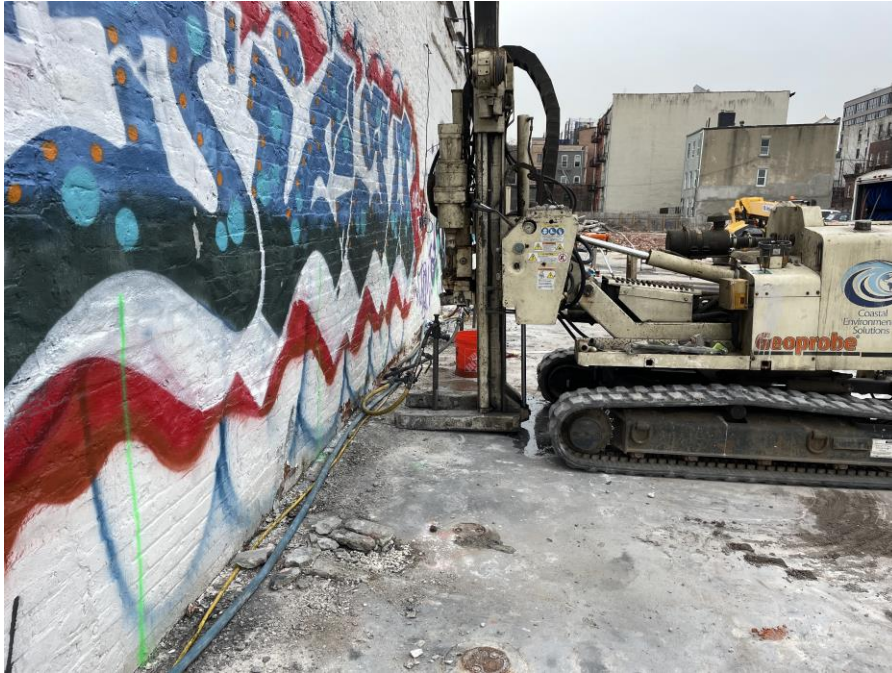
Photo 1: Regensis applying remedial products at injection point IP27 (facing east).
