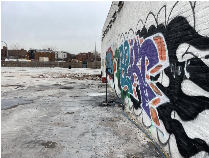
Photo 2: Regensis applying remedial products at injection points IP22(facing west).
