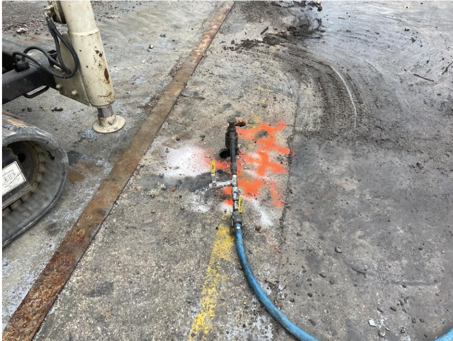
Photo 1: Regensis applying remedial products at injection point IP37A (facing northeast).
