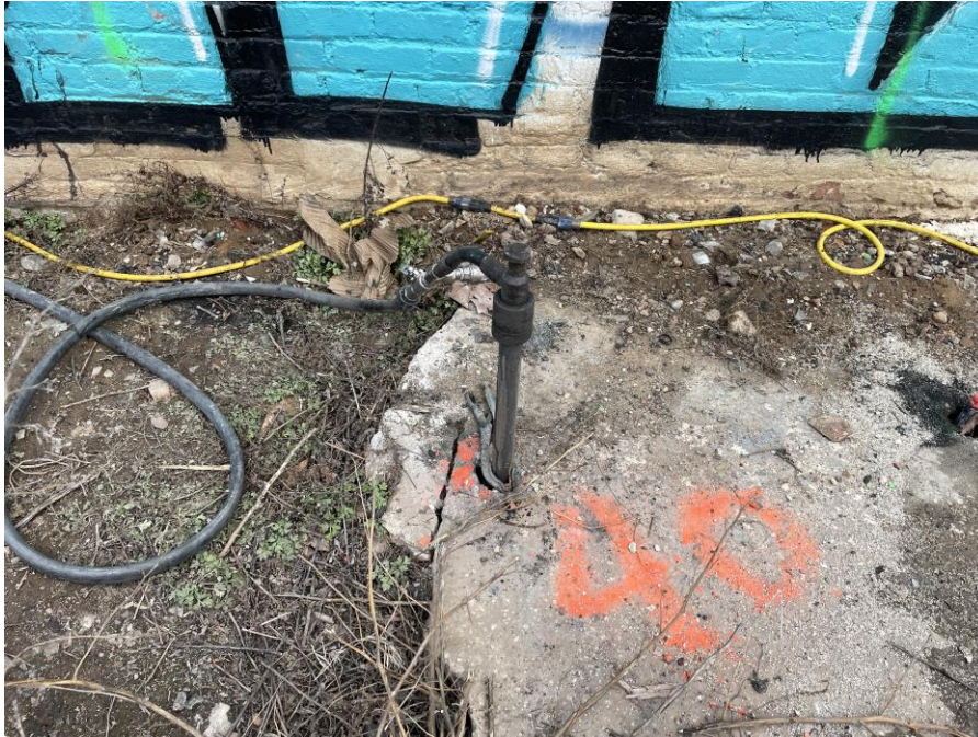
Photo 1: Regensis applying remedial products at injection point IP40 (facing north).
