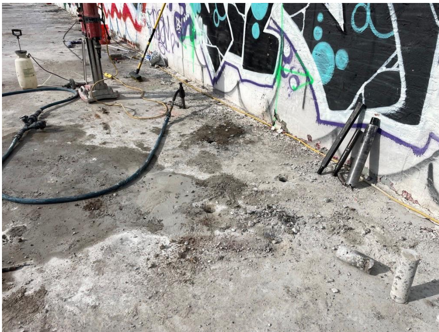
Photo 2: Regensis applying remedial products at injection point IP30 (facing northwest).
