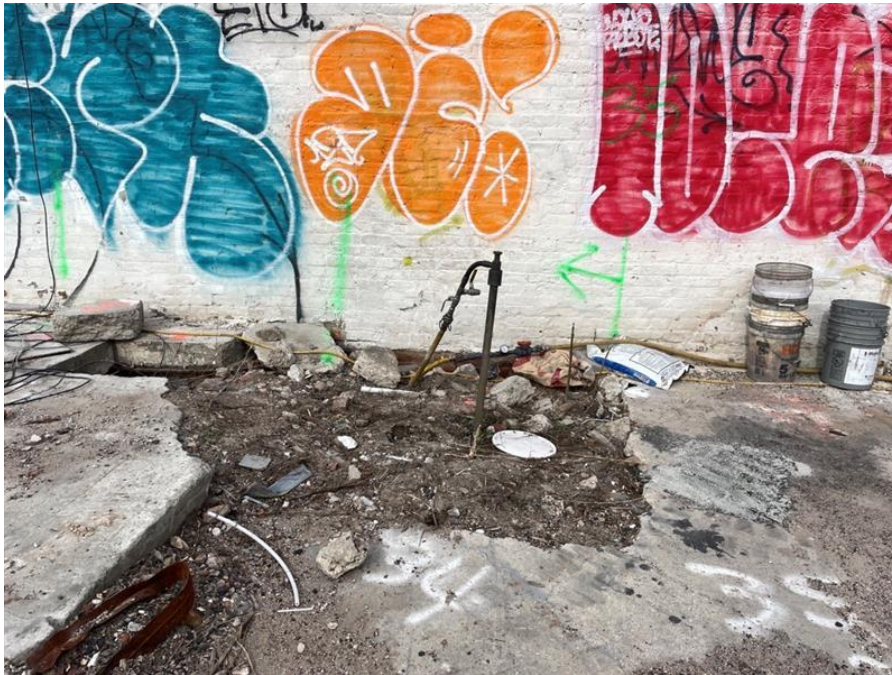
Photo 1: Regensis applying remedial products at injection point IP35 (facing north).
