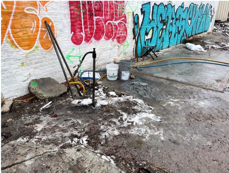
Photo 1: Regensis applying remedial products at injection point IP35 (facing northeast).
