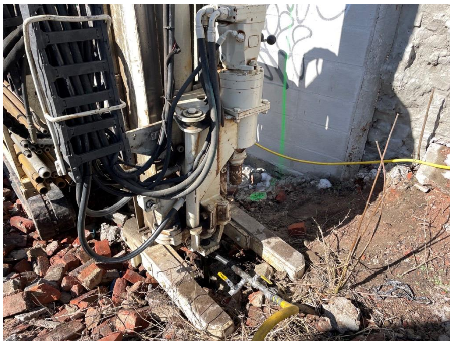
Photo 1: Regensis applying remedial products at injection point IP45 (facing southwest).
