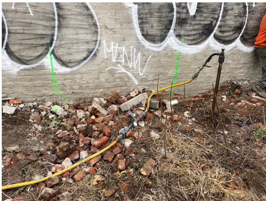
Photo 2: Regensis applying remedial products at injection point IP48 (facing northwest).
