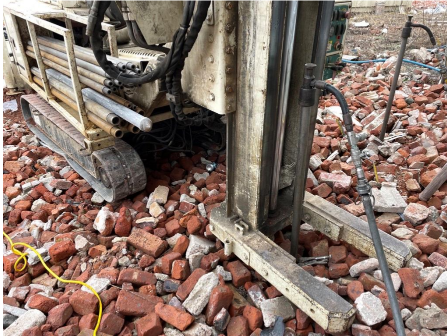
Photo 1: Regenesis applying remedial products at injection point IP51 (facing south).
