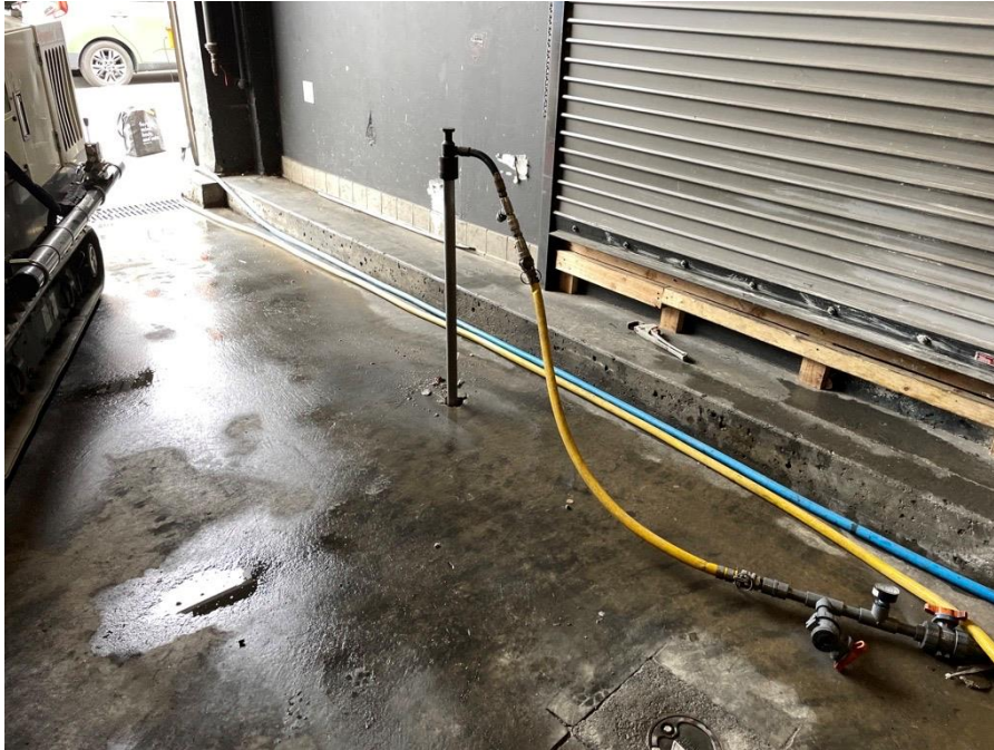
Photo 1: Regensis applying remedial products at injection point IP02B (facing northeast).
