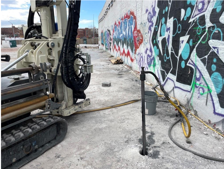
Photo 1: Regenesis applying remedial products at injection point IP31 (facing northwest).
