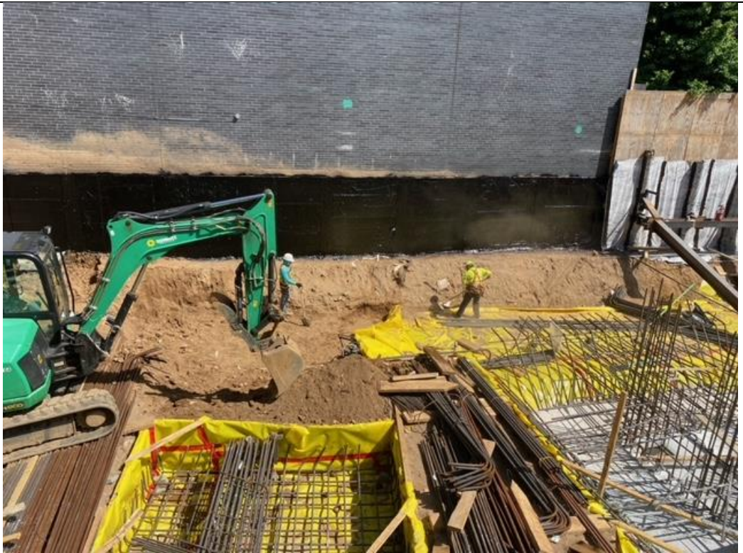
Photo 1 – Facing North Soil grading and rebar work along northwestern corner of the Site.
