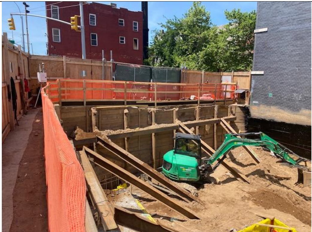
Photo 4 – Facing West CAMP 1 station located in southwest corner of Site.
