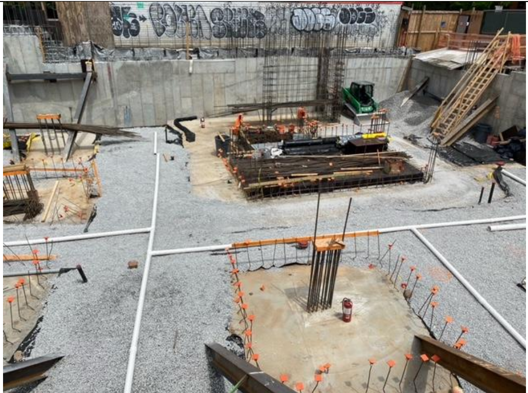
Photo 4 – Facing South Continue placing SSDS piping throughout the Site
