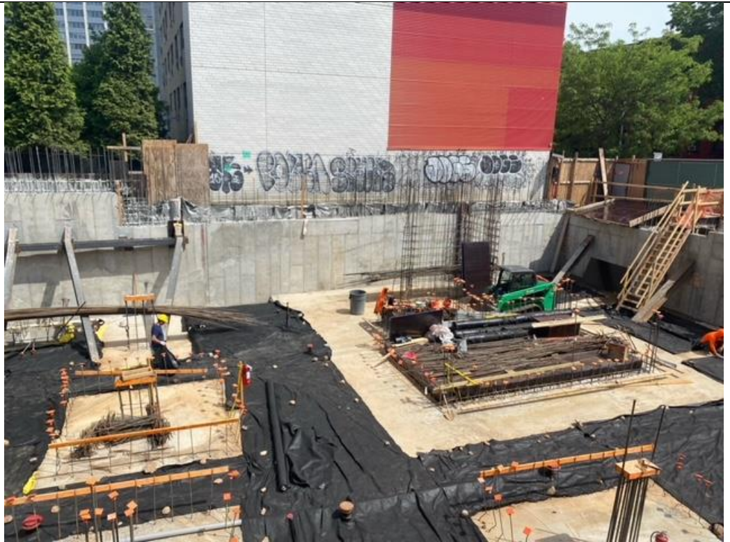
Photo 4 – Facing North Laying down base layer of geotextile fabric for SSDS.
