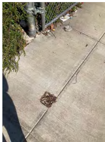
Photo 12: View of cover for shut-off valve for water located directly outside of entrance to subject site.
