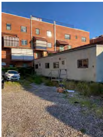
Photo 3: View of trailer located in the northern portion of the site.
