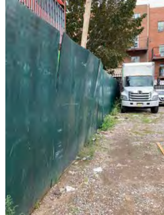
Photo 14: View of barrier between the subject site and adjacent construction site.
