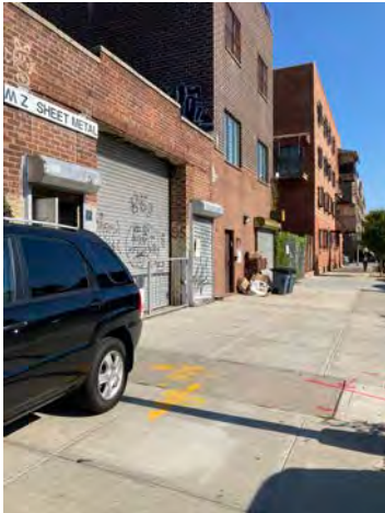
Photo 9: View of adjacent warehouse to the northeast labeled "MZ Sheet Metal".
