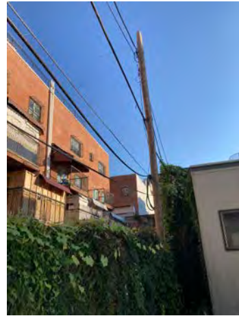
Photo 8: View of powerlines overhead along rear of the property.
