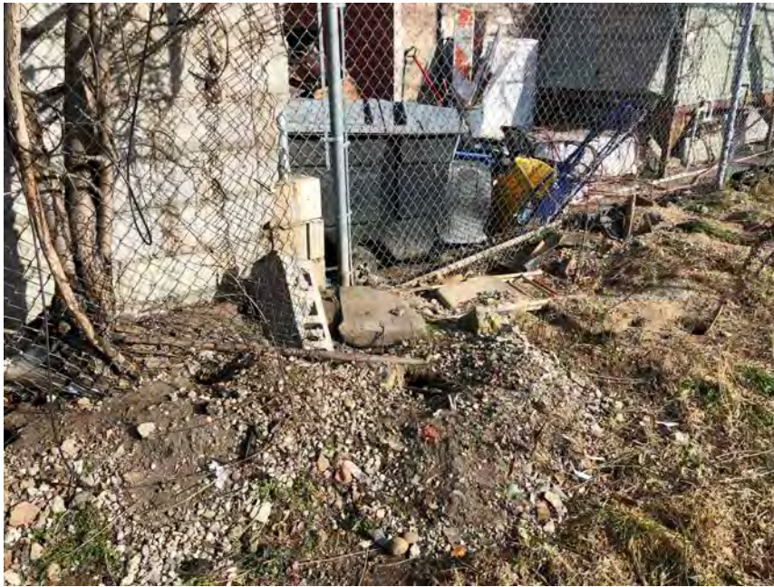
5. Typical on-site demolition debris
