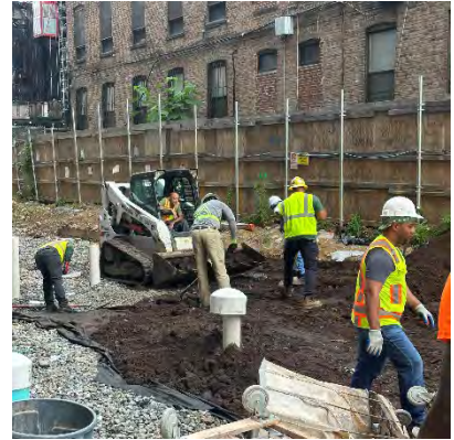
Placing engineered cover soil over geofabric material
