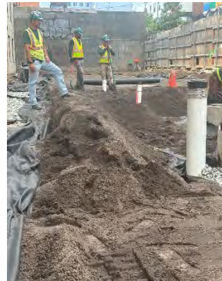
Placing and grading engineered soil
