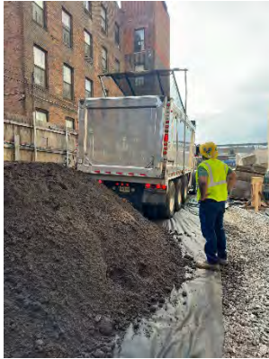
Delivery of engineered cover soil
