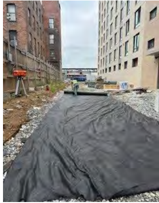
Placing geotechnical fabric over stone
