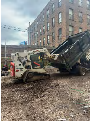
Off loading crushed stone for base course under stepping stones
