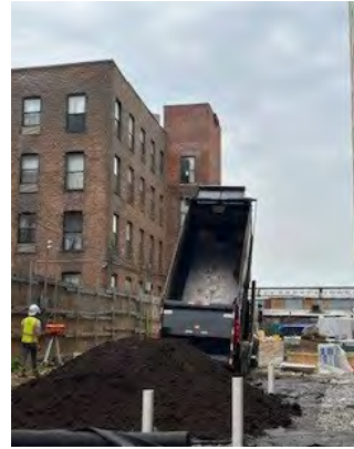
Placing engineered soil over geotechnical fabric
