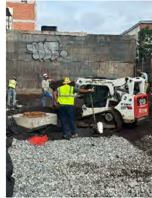
Placing and grading engineered cover soil
