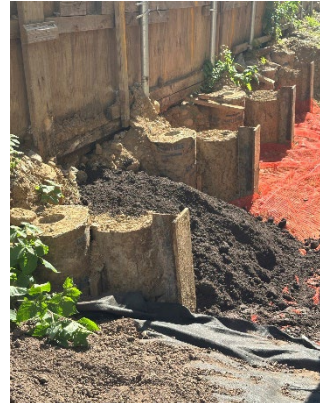
Placing planting soil over demarcation material
