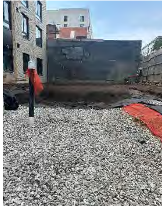
Engineered cover soil at the west end of the courtyard
