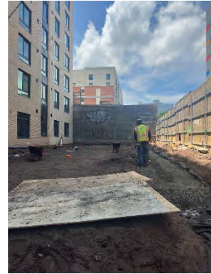
Installing crushed stone base layer
