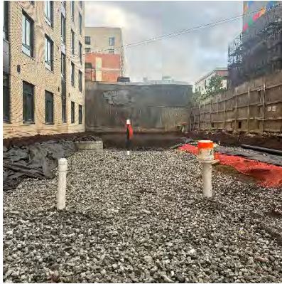
Engineered cover soil at the west end of the courtyard
