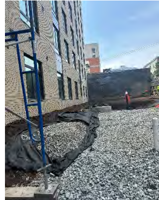
Engineered cover soil along the building
