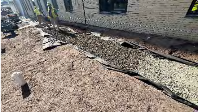
Placing stone base over geotechnical fabric for steppingstones
