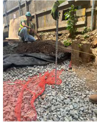
Measured thickness (> 2 ft.) of proposed soil cover over stone along north property line
