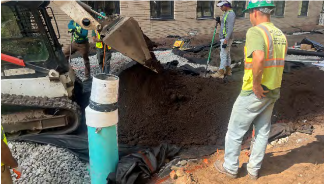
Placing engineered soil over geo-fabric
