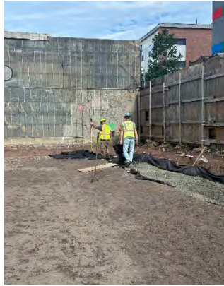
Installing Item 4 for base under steppingstone walkway
