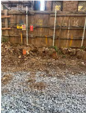
Existing soil excavated to allow for 2' of clean fill
