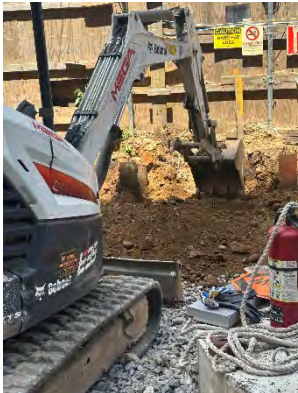
Excavating existing soil to allow for 2' clean soil cover
