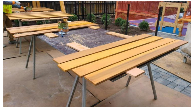
8. Wood staining and painting at rear courtyard
