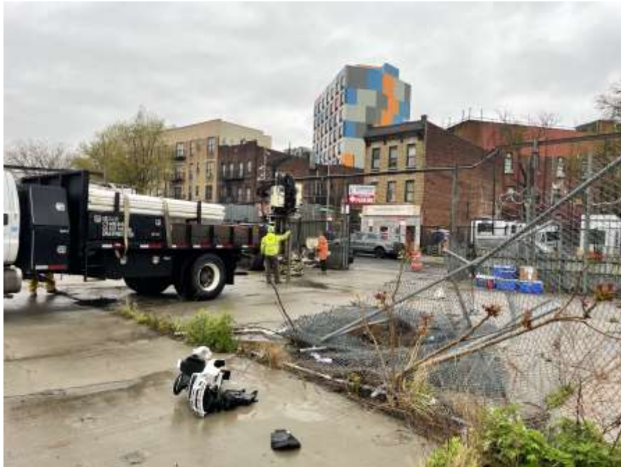
Photo 1: View AARCO advancing SB11 (facing northwest).
