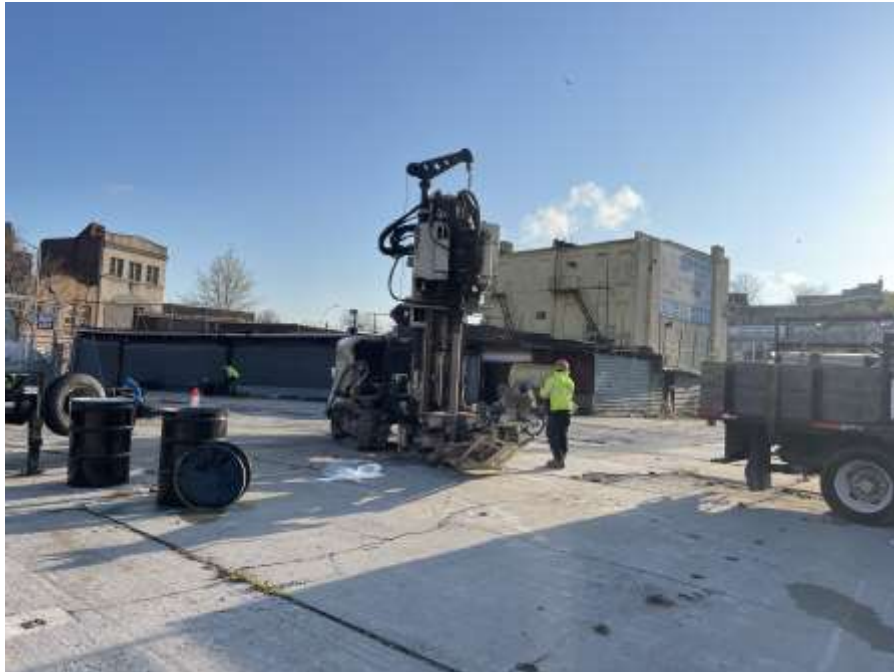
Photo 1: View AARCO advancing SB14 (facing northeast).
