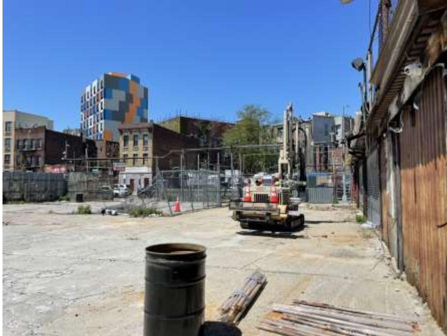
Photo 1: AARCO advancing SB06_W (facing north).
