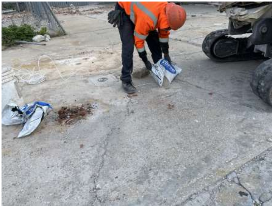
Photo 2: AARCO installing soil vapor monitoring point SVP06 (facing northwest).
