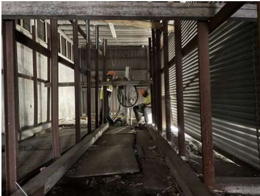
Photo 1: AARCO advancing soil boring SB06R (facing south).
