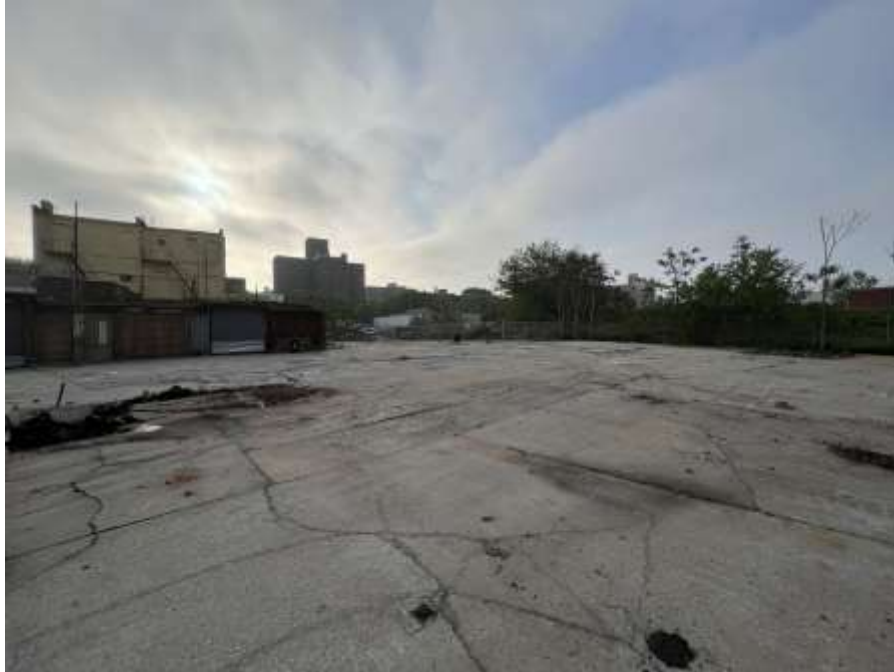
Photo 1: General view of the site at the beginning of the day (facing south).
