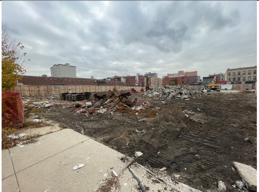
Photo 4 – View of stockpiling of mixed masonry material and concrete.
