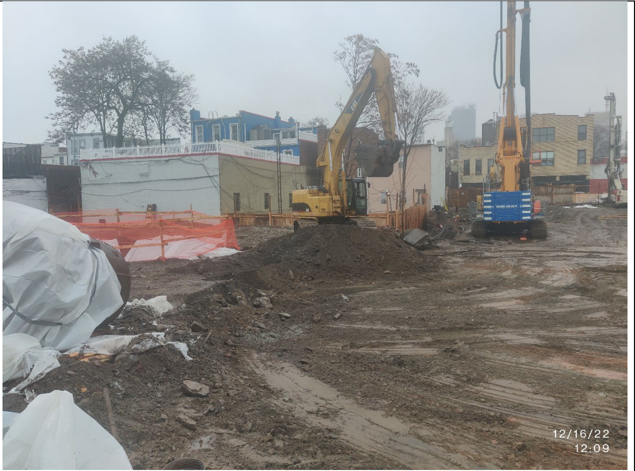
Photo 5 – Representative view of material from WC-2 being loaded for off- site disposal at Conestoga.
