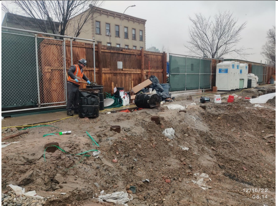
Photo 3 – Representative view of drum removal.
