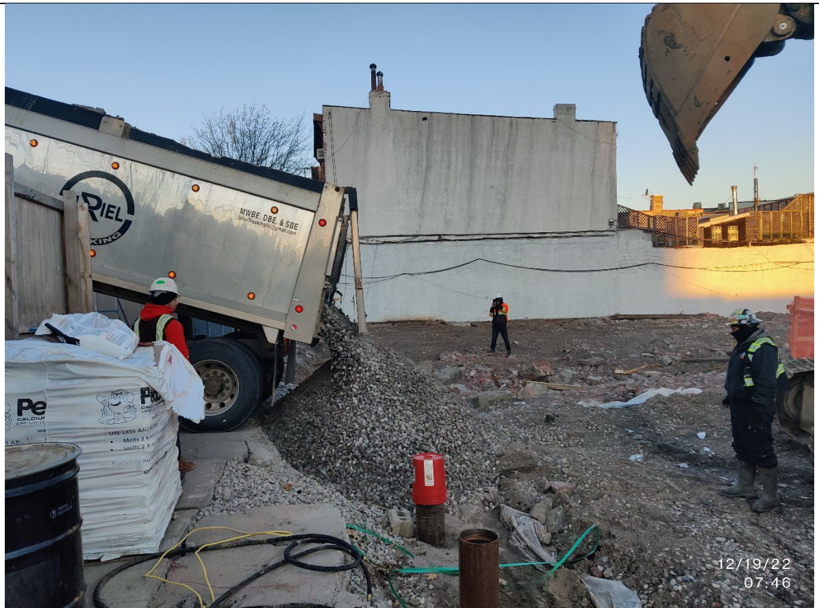
Photo 2 - Stone delivery for trucking pad at Sie entrance/exit at WC-2
