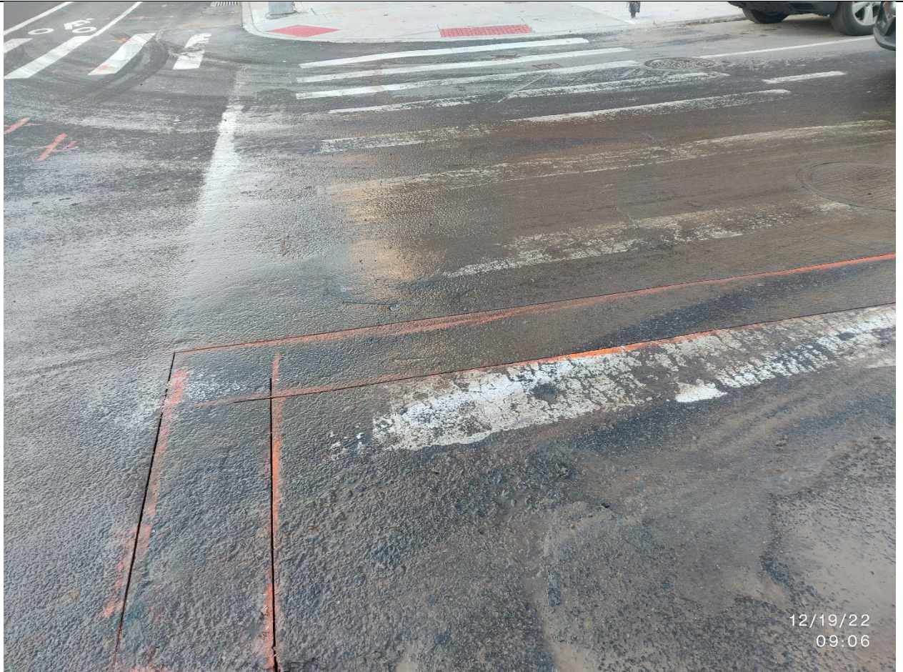
Photo 7 – Saw cutting work that generated soil/ dirt by national grid directly outside the site and in the street (intersection of union and 3 rd avenue)
