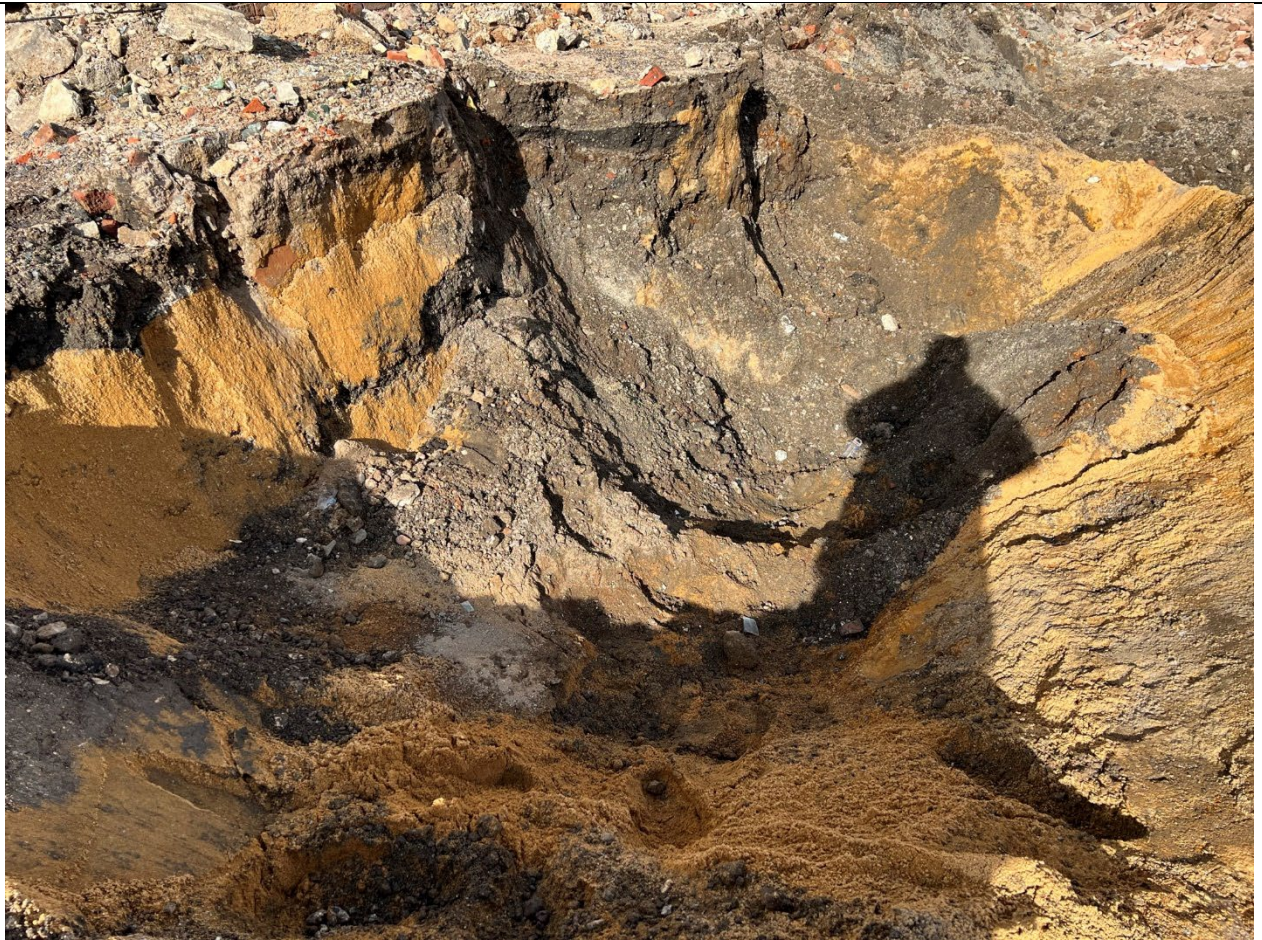
Photo 5 – Photo of the tank bed of Tank 3, where endpoint and sidewall samples were collected.
