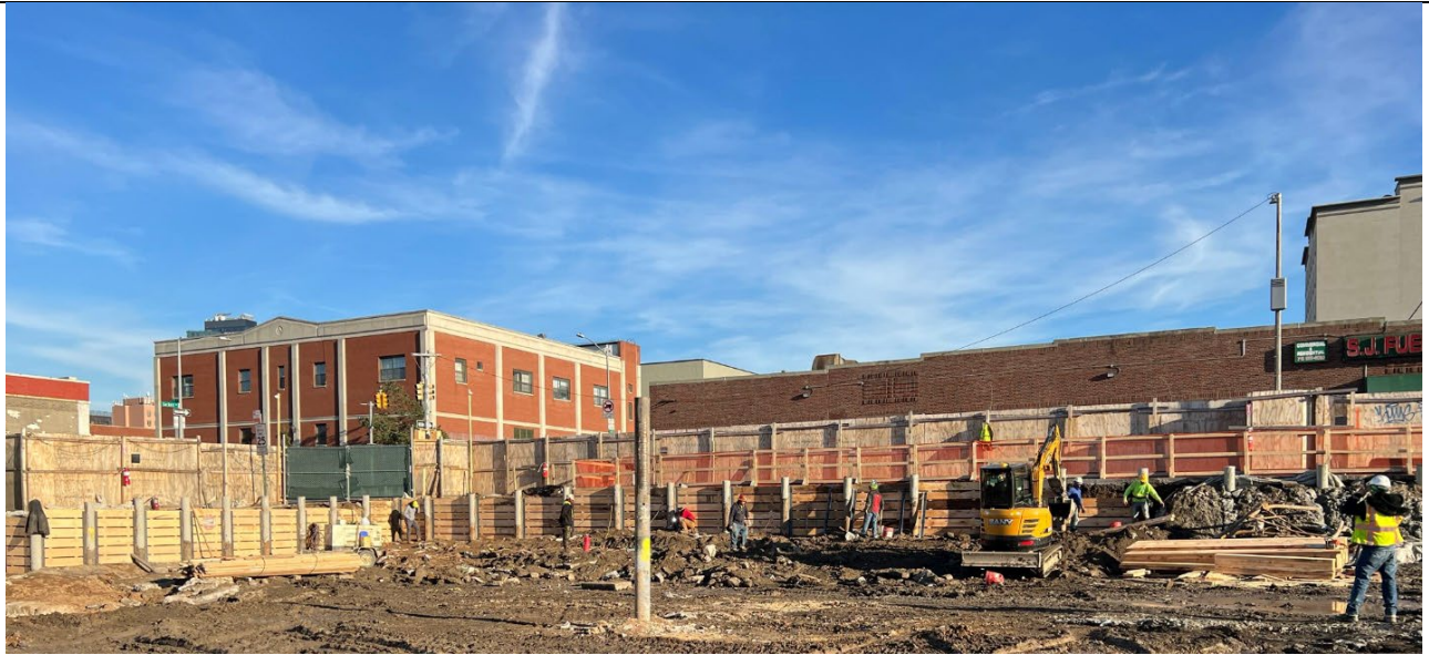
Photo 4 – Representative photo of workers installing lagging.
