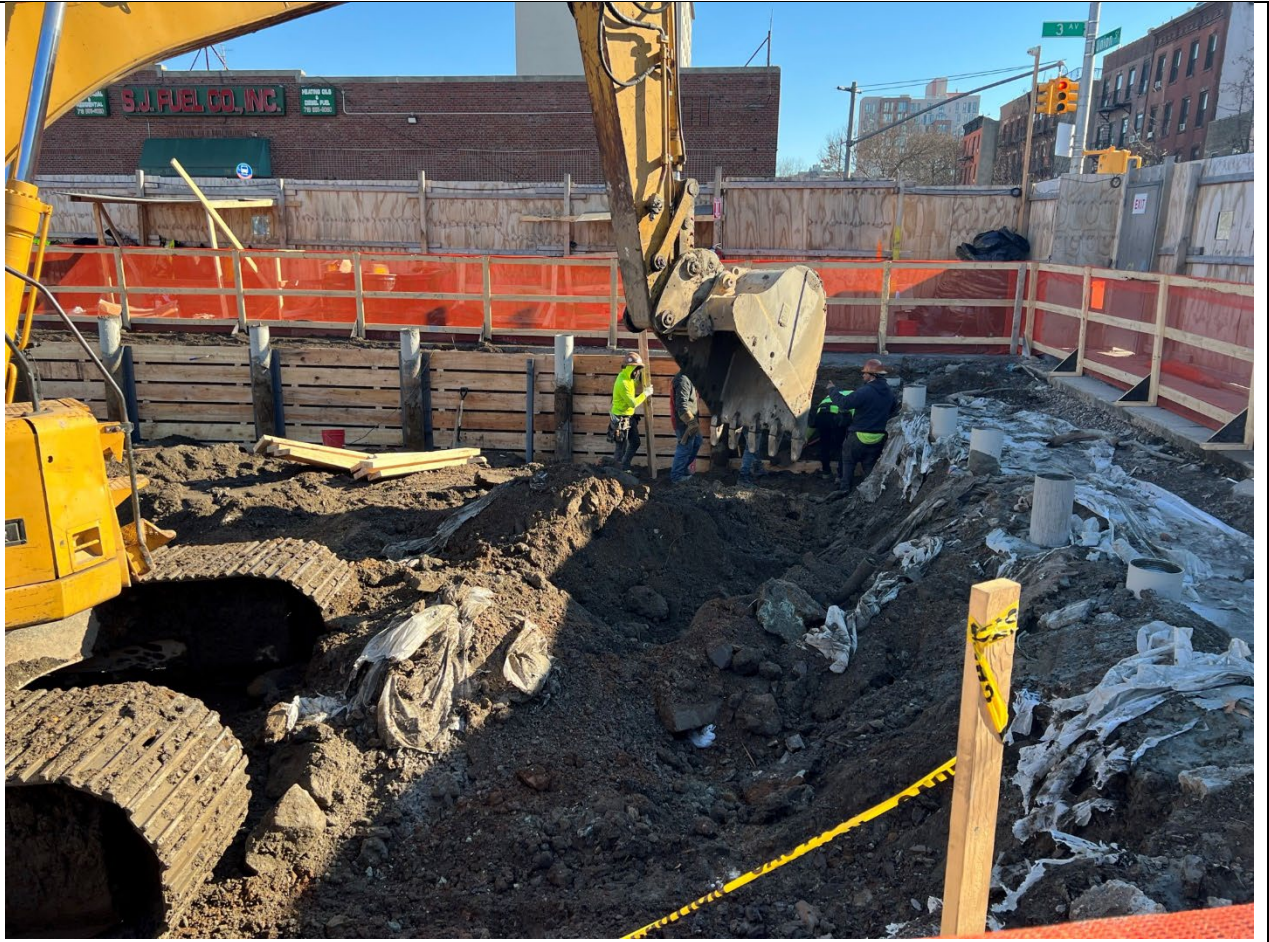
Photo 4 – Representative photo of workers installing lagging.
