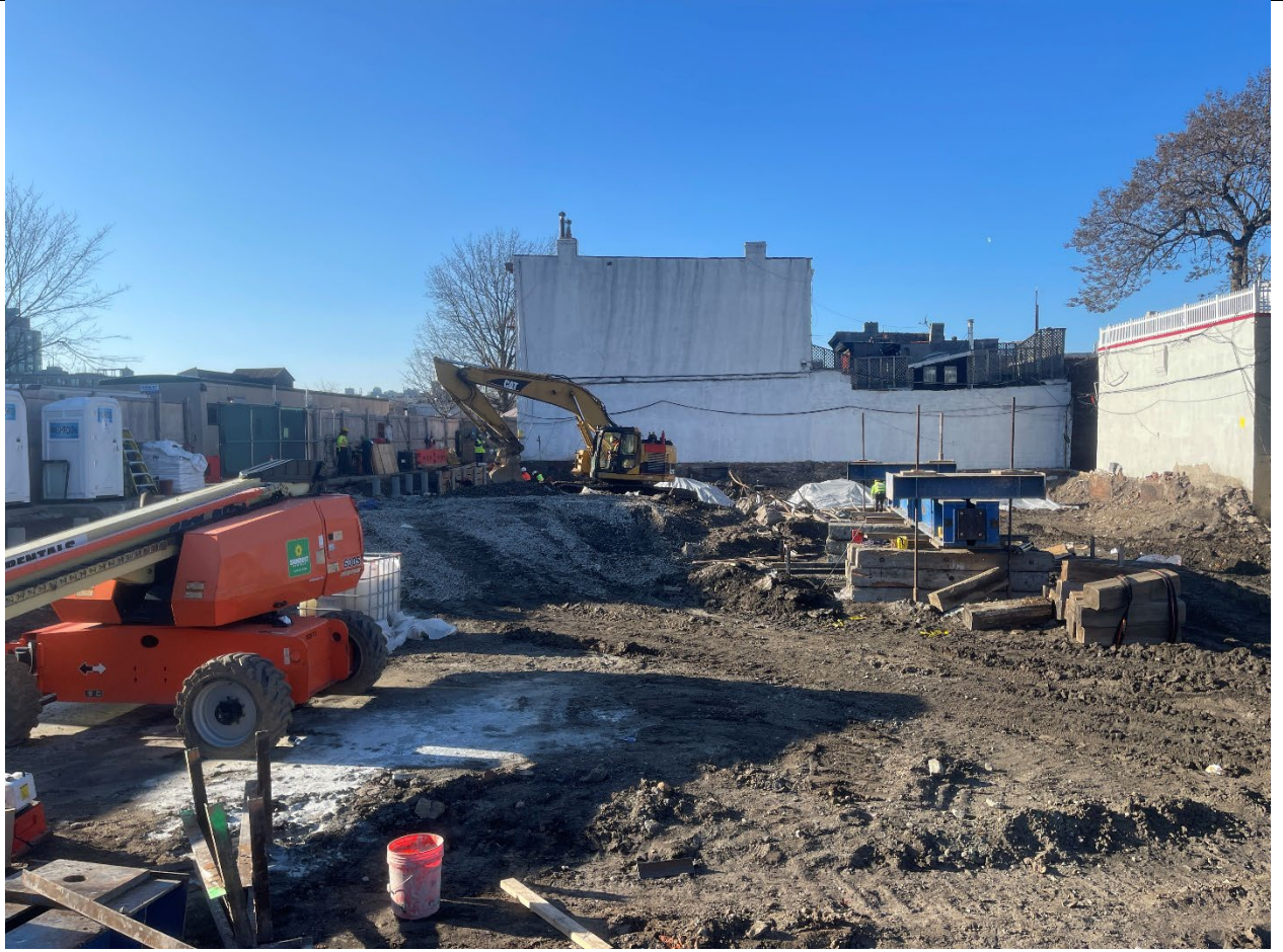
Photo 5 – Continued pilling work along union street.
