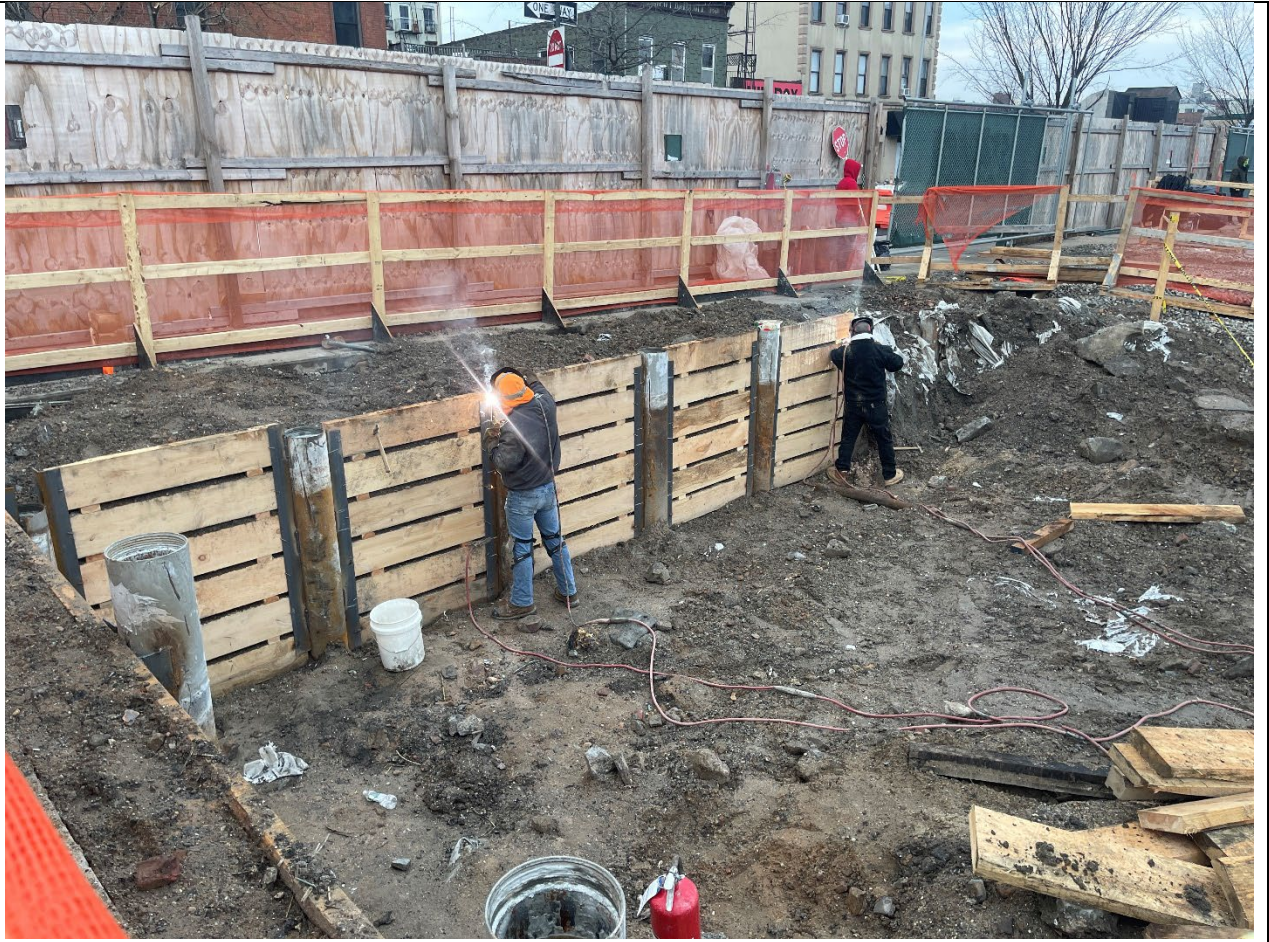
Photo 2 – Welding and piling work along Union Street.
