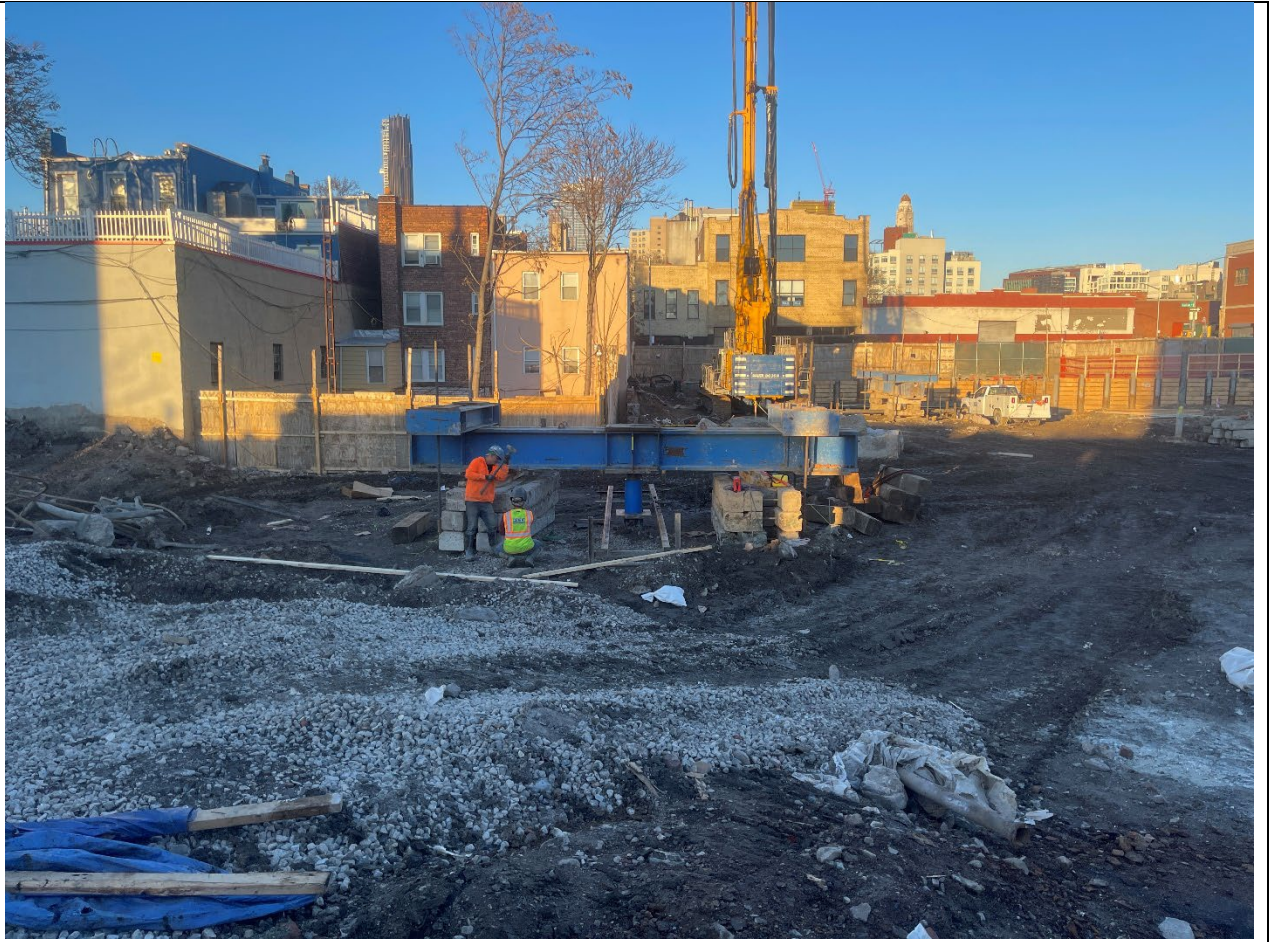
Photo 4 – Set up for compression and load testing.
