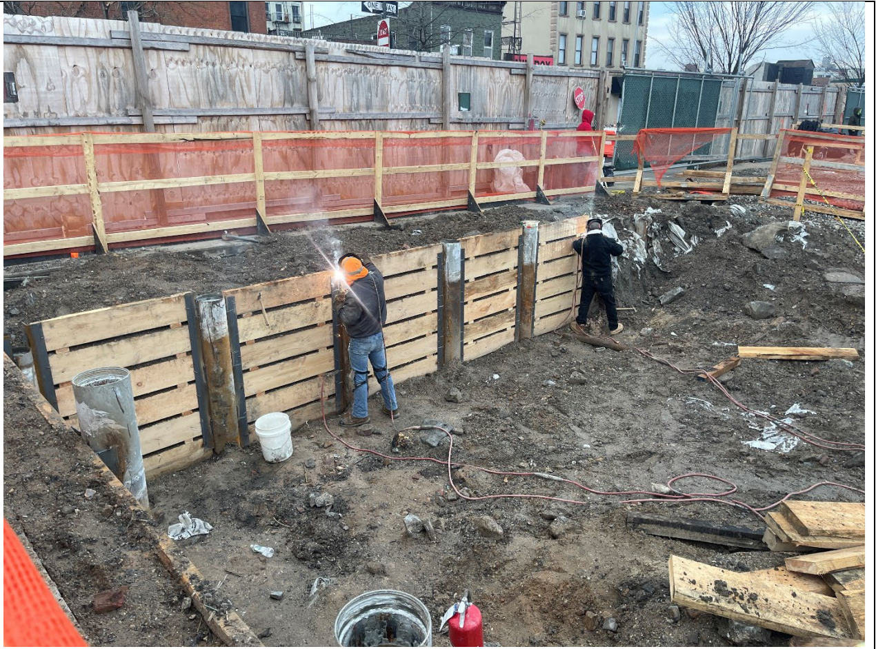
Photo 2 – Representative view of welding and piling work along Union Street.
