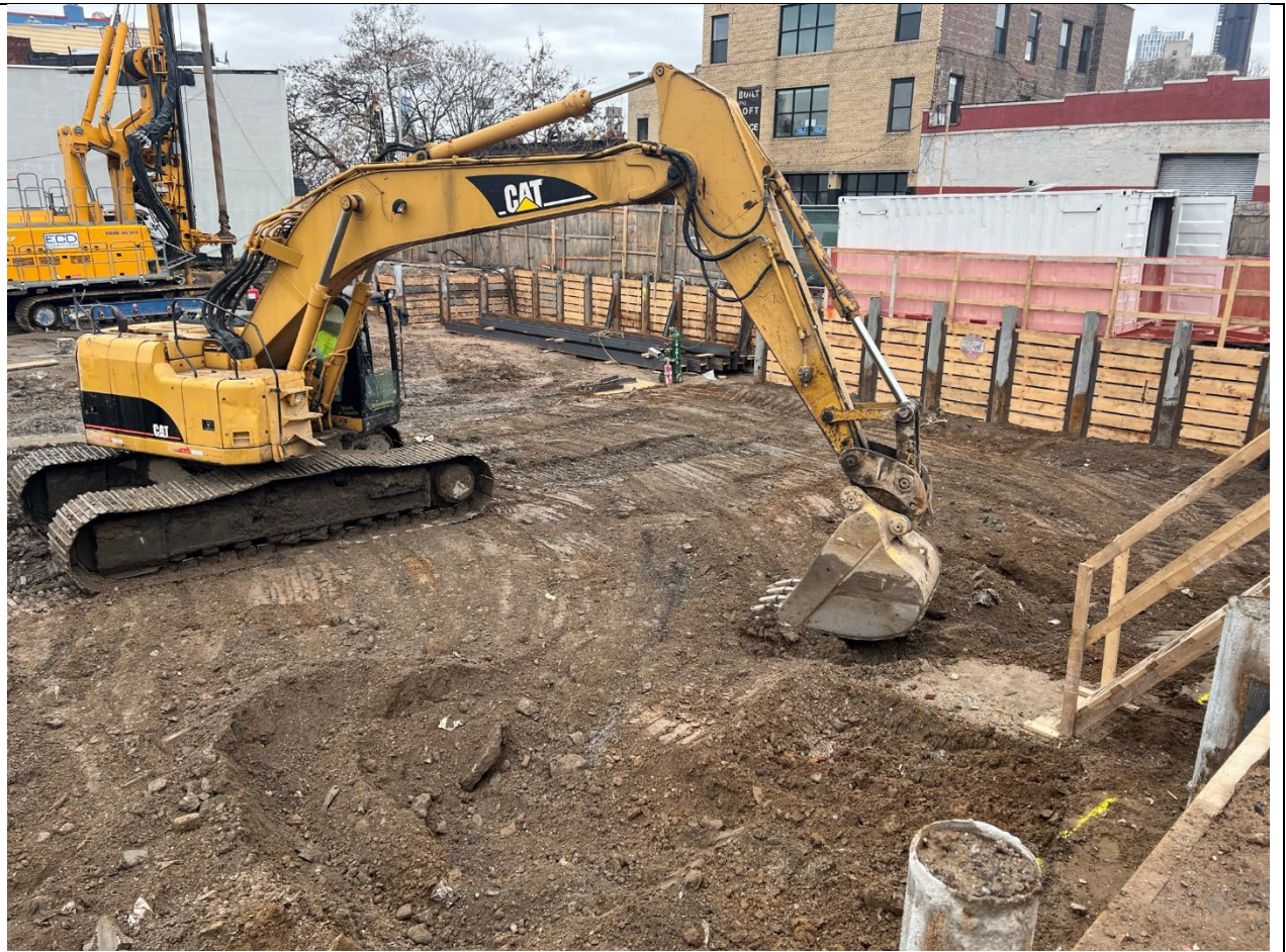
Photo 3 – WC-8 being graded for the pile machine.
