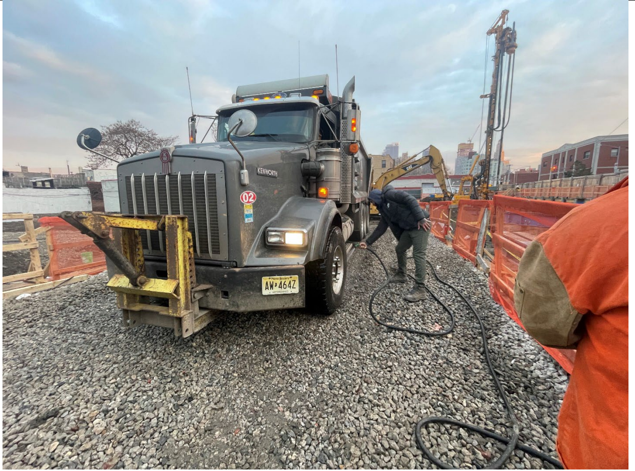
Photo 5– Representative view of truck wash on tracking pad.
