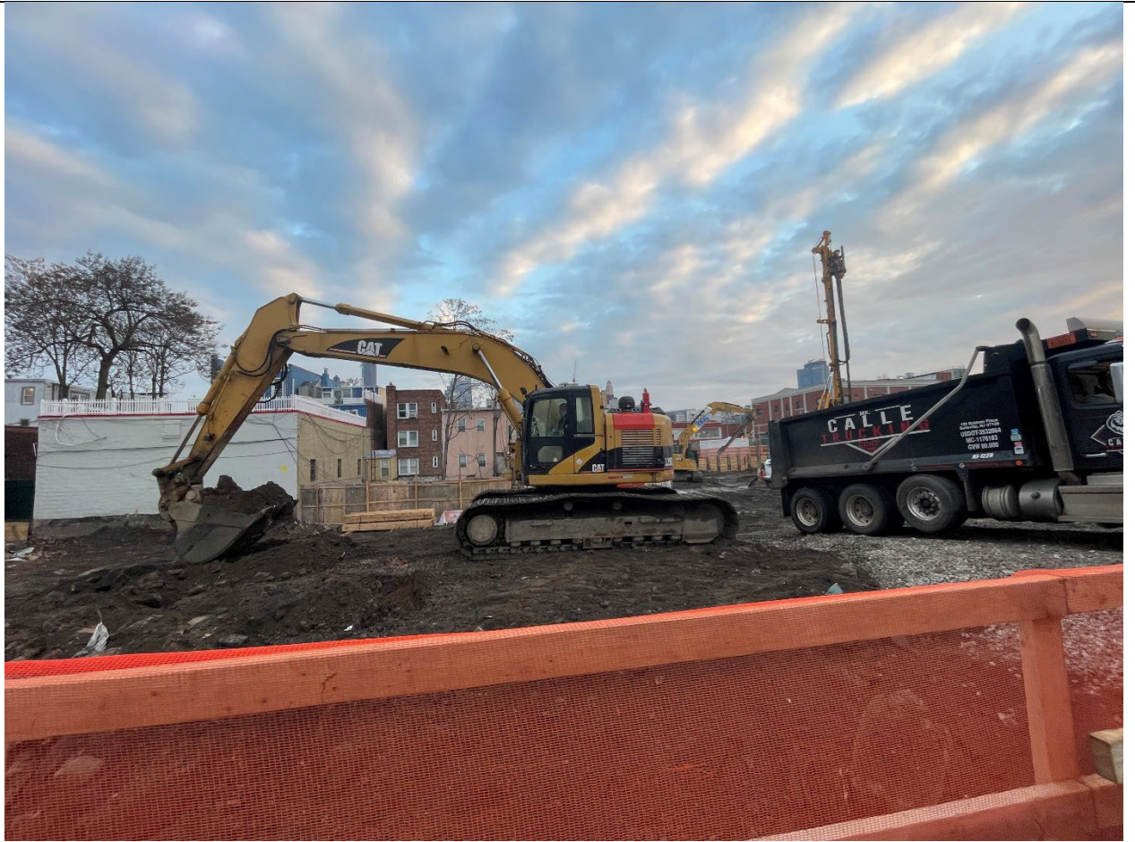
Photo 4 – Additional view of hotspot stockpile loadout from WC-2.
