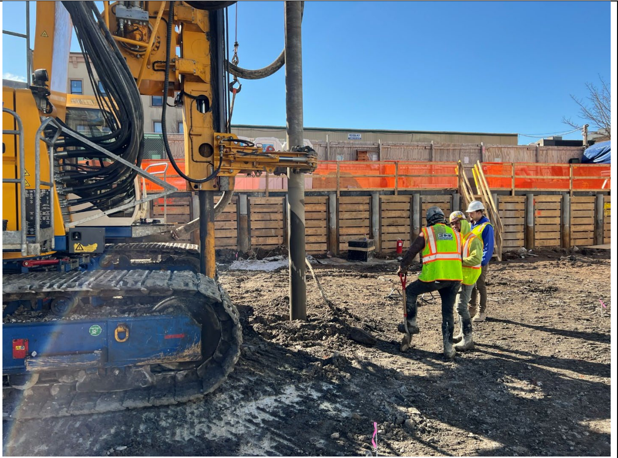
Photo 3 – Representative photo of EDC installing piles.
