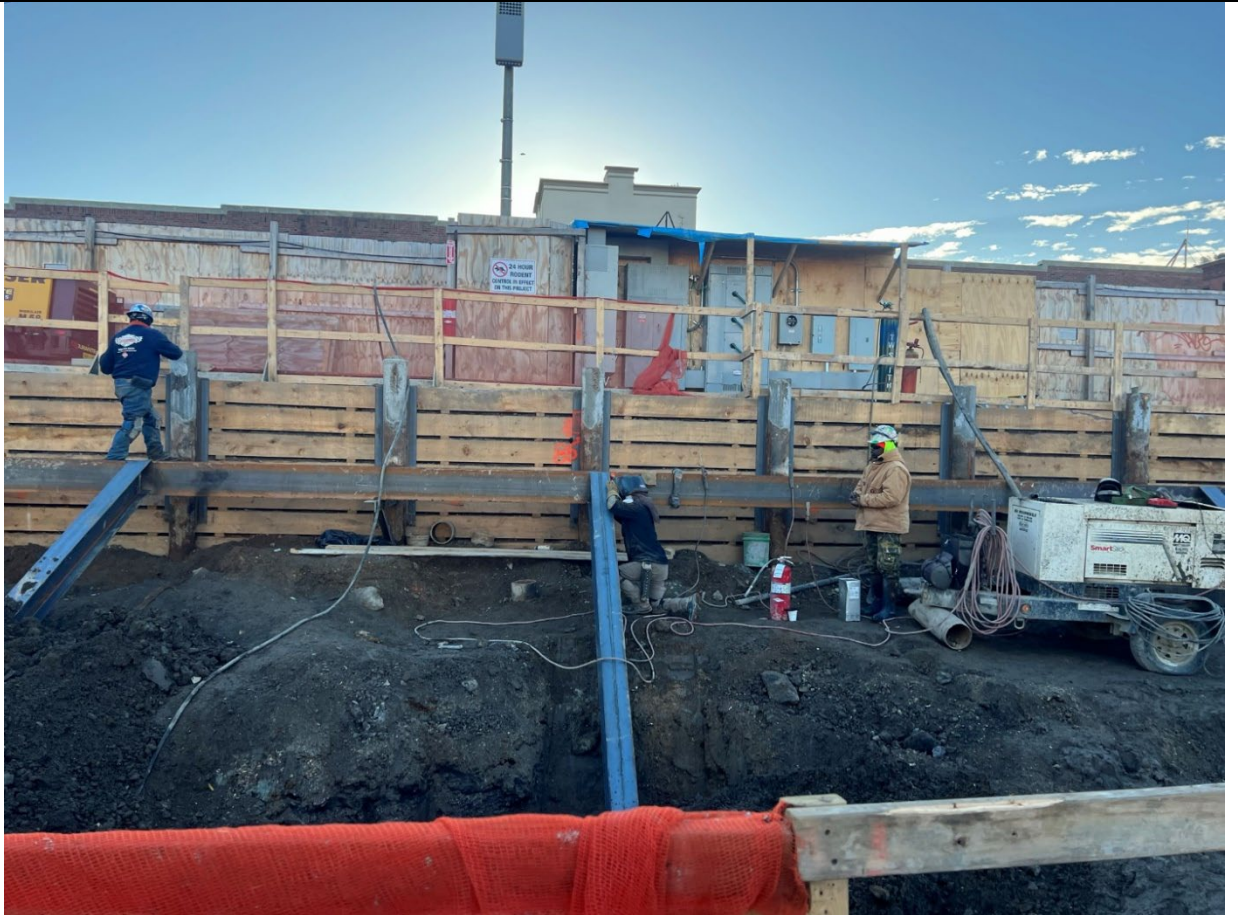
Photo 2 – Representative photo of workers welding whalers along 3 rd Avenue.
