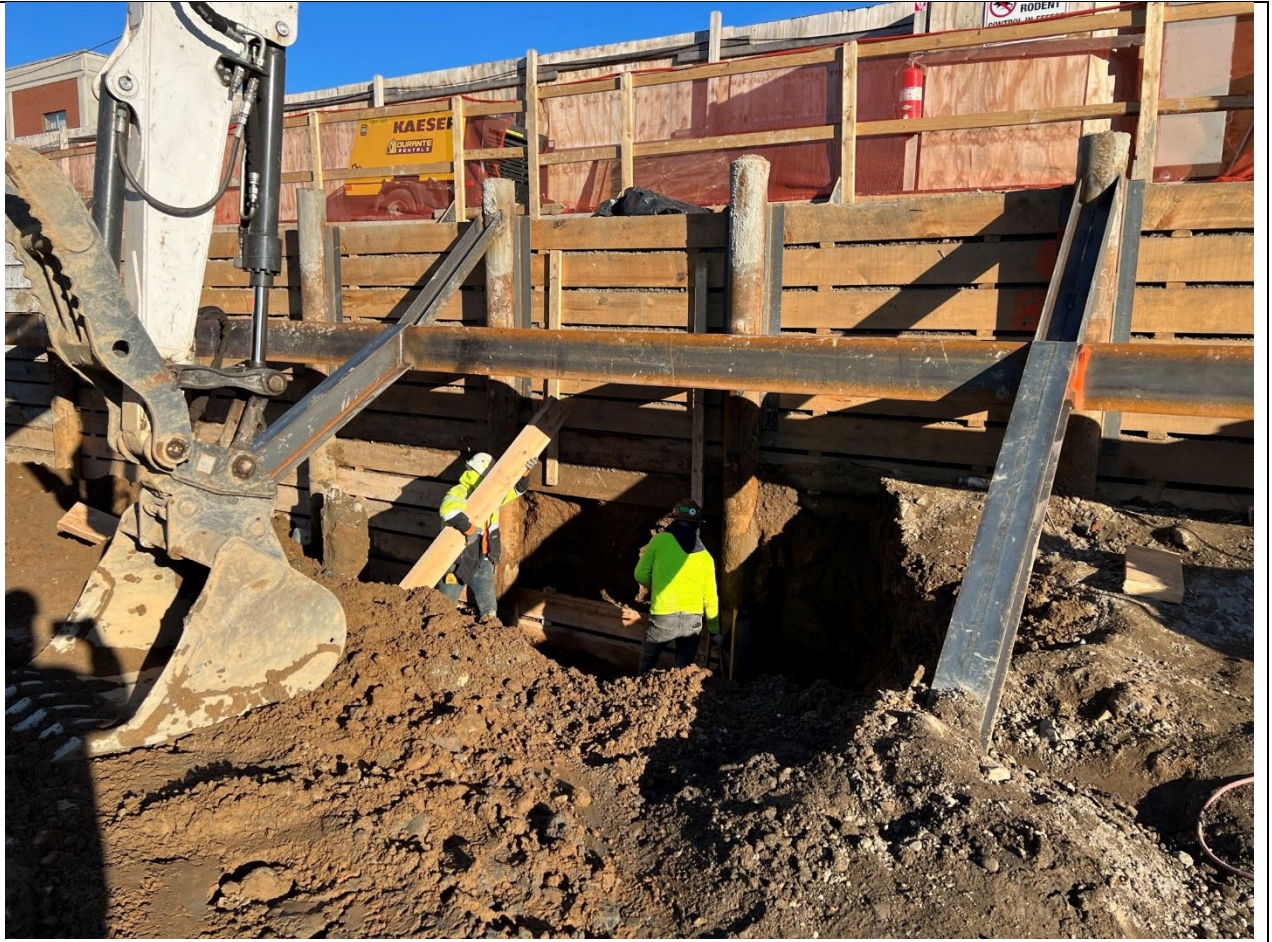
Photo 4 – Representative photo of lagging along 3 rd Avenue.
