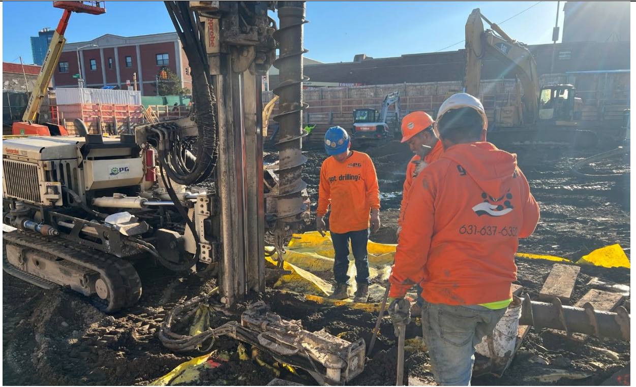
Photo 1 – Representative photo of auguring hot spot SB-14.
