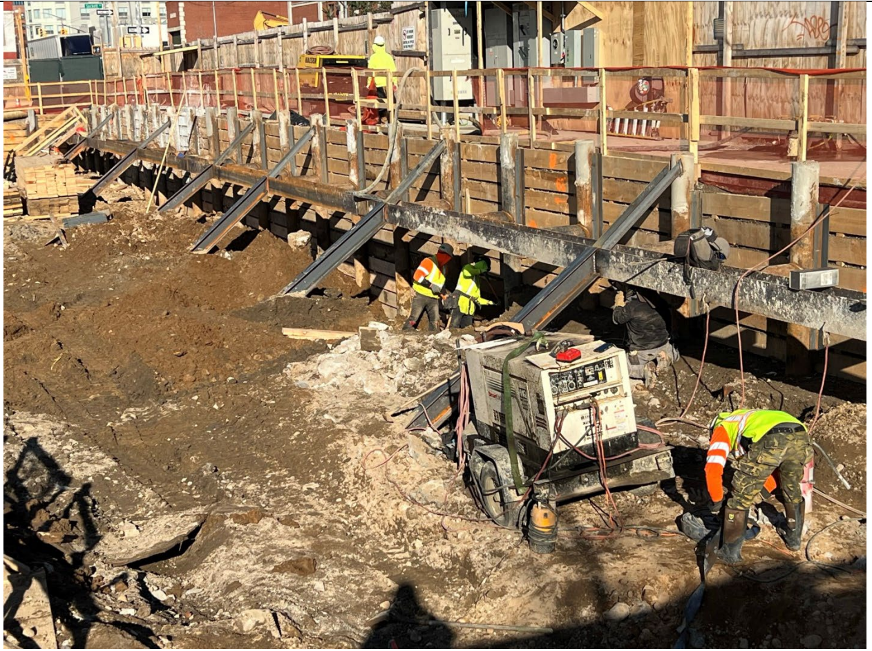
Photo 4 – Representative photo of lagging along 3 rd Avenue.
