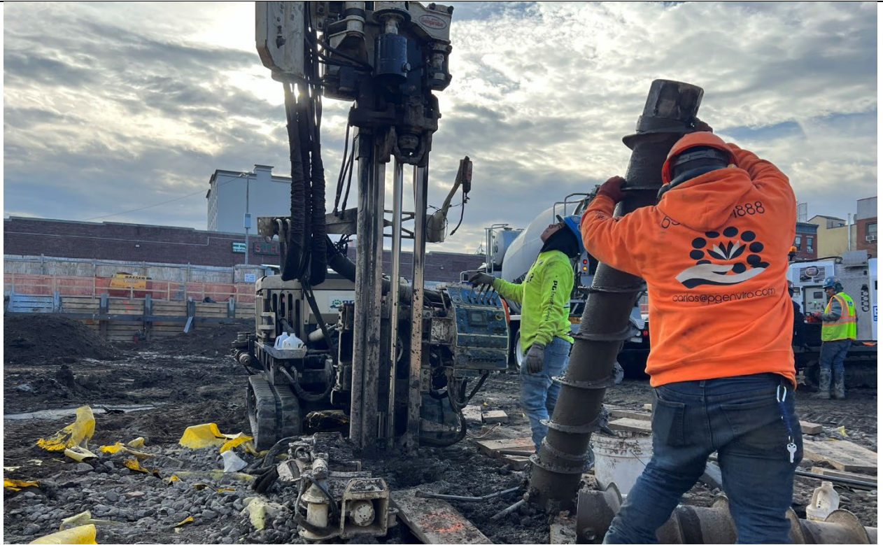
Photo 1 – Representative photo of auguring hot spot SB-14.
