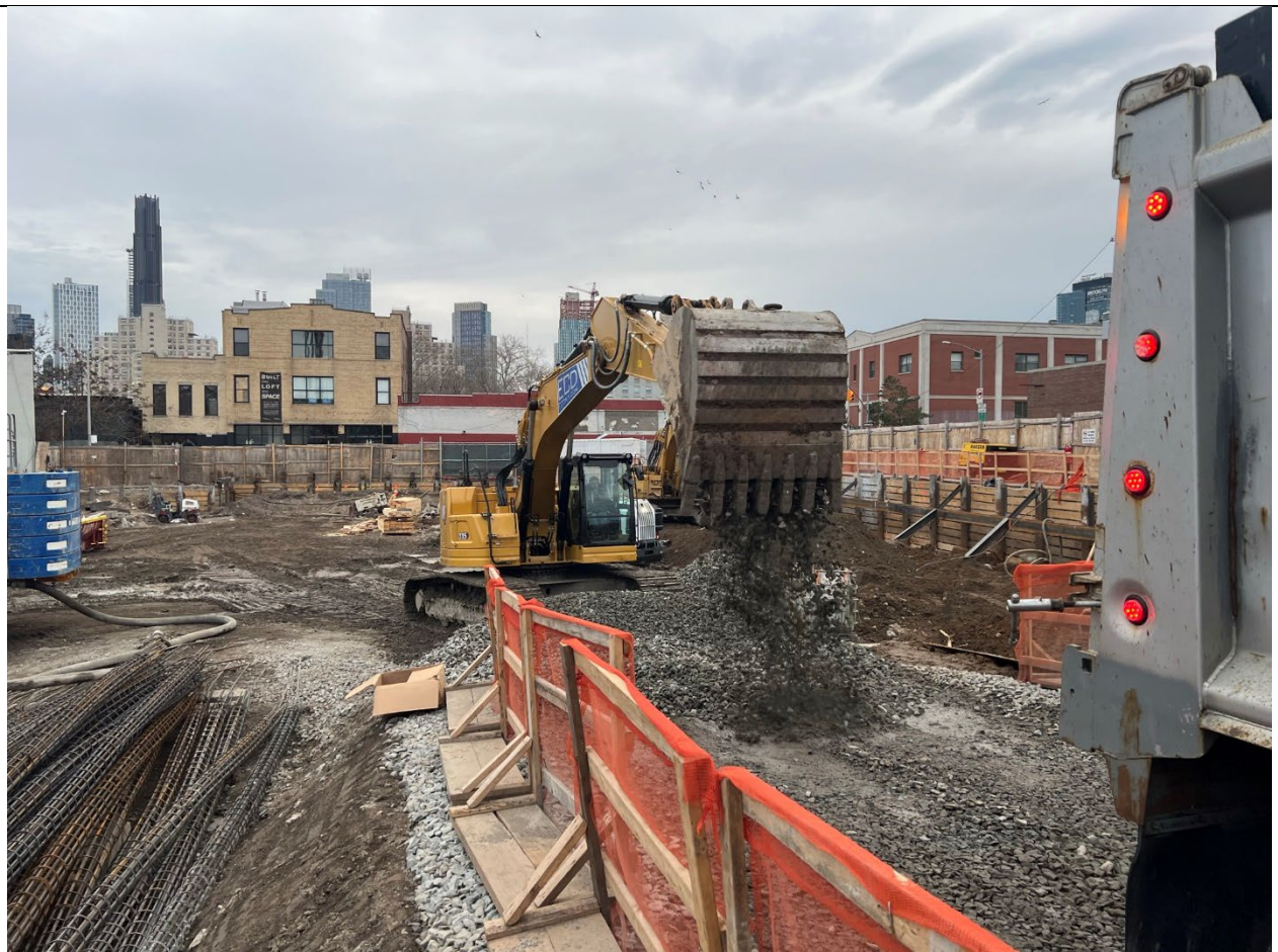
Photo 2 – Representative photo of adding new stone to track pad delivered to site today.
