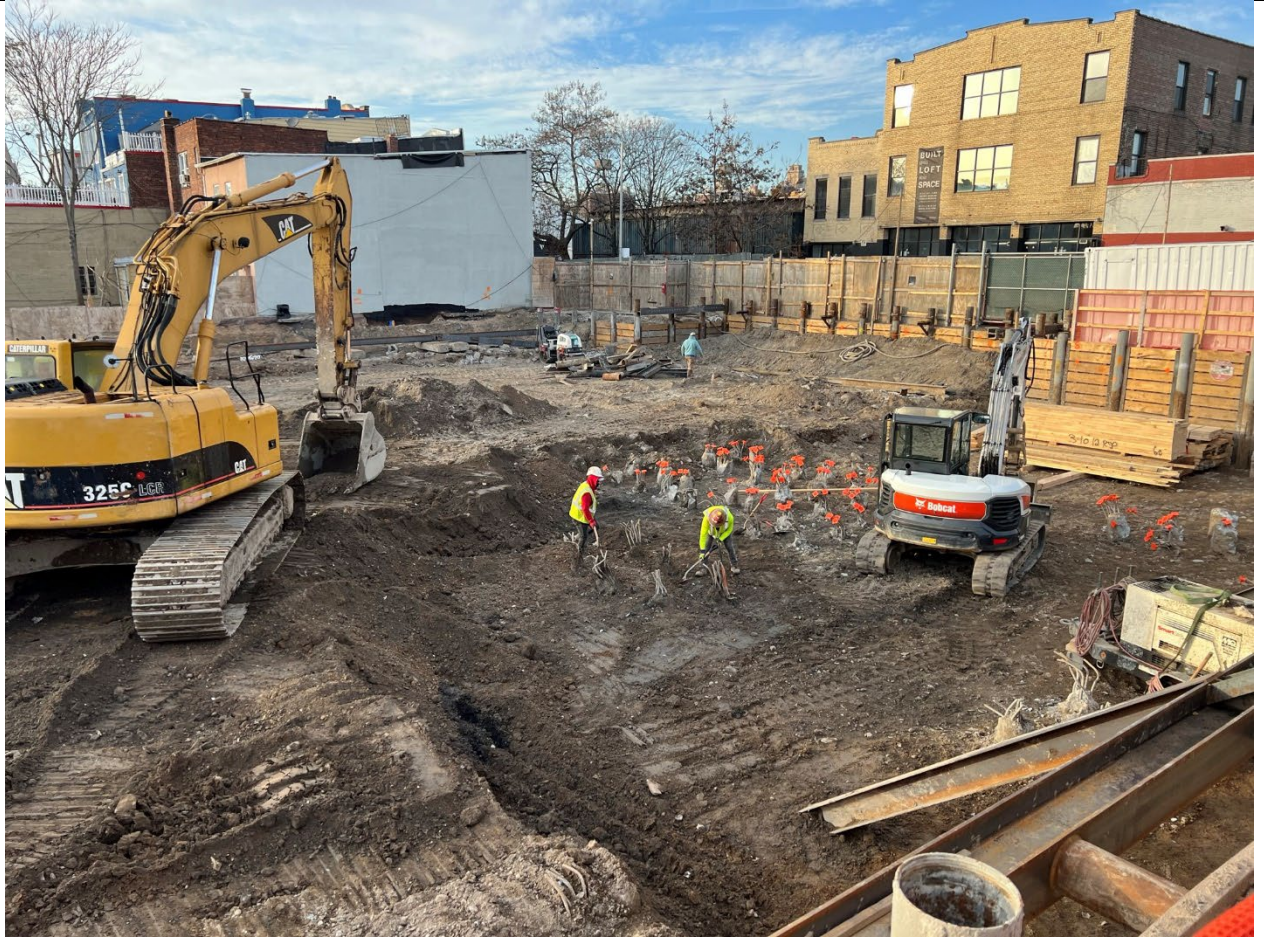
Photo 3 – Representative photo of exposing installed piles.
