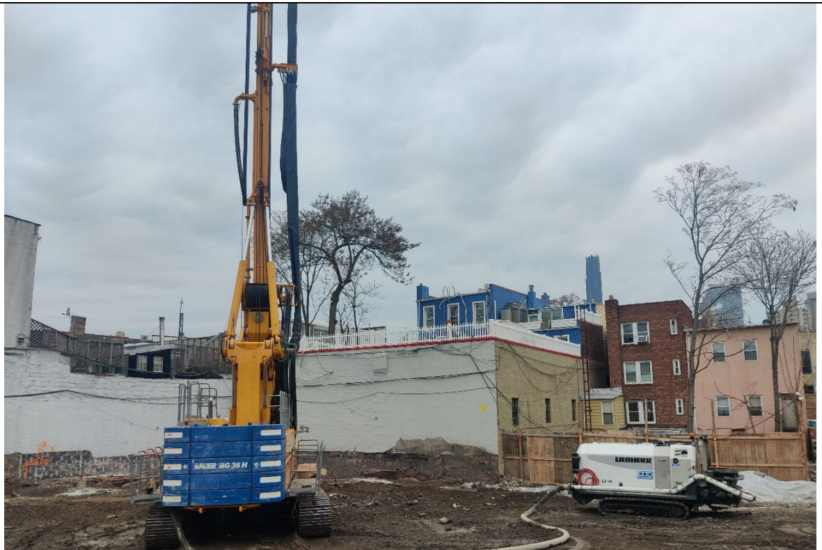
Photo 2 – Representative view of EDC installing a pile.
