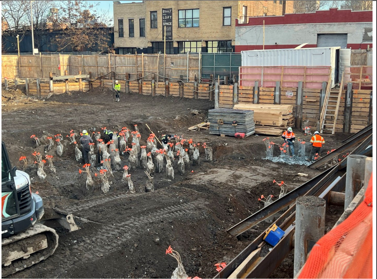
Photo 3 – Representative photo of exposing piles in WC-8.
