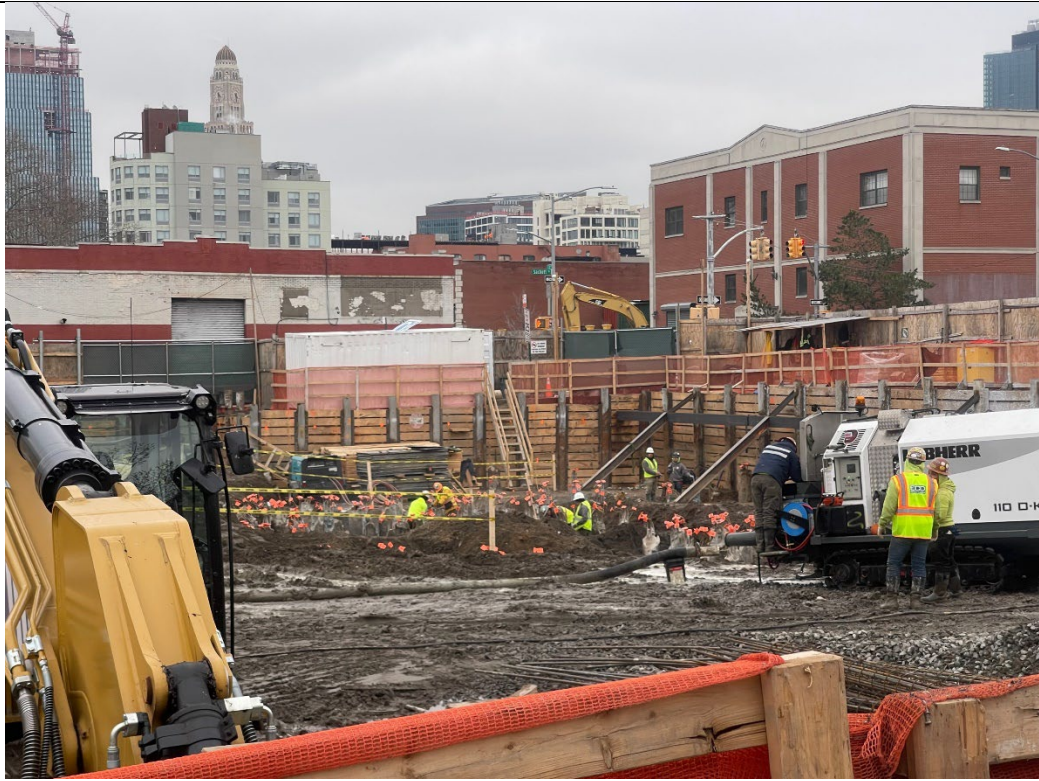
Photo 4 – Representative photo of removing grout from piles in WC-8.
